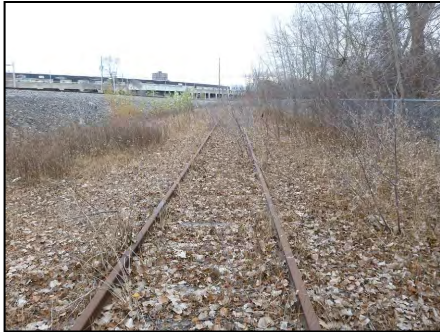
Image 17. The abandoned CPR spur line to the southwest of the O-Train line, facing southeast. (PR15-41D001) Note the limited space between the track and the active rail corridor boundary fence.
