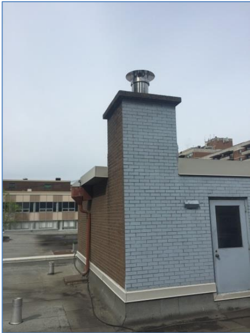
Photo 2. 385 Slater St. rooftop
