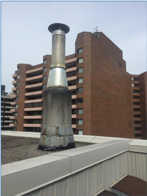
Photo 3. 400 Albert St rooftop
