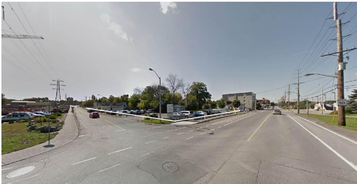
/ Figure 1: View of intersection at Scott Street and McRae looking west.
