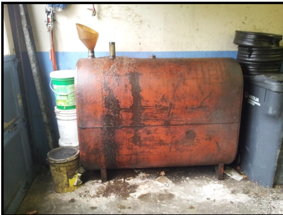
Photograph 8: View of the waste oil AST on east wall of Gifford Automotive garage unit. Photograph depicts staining around AST, absorbent material on and around the AST and recent oil releases to the floor.
