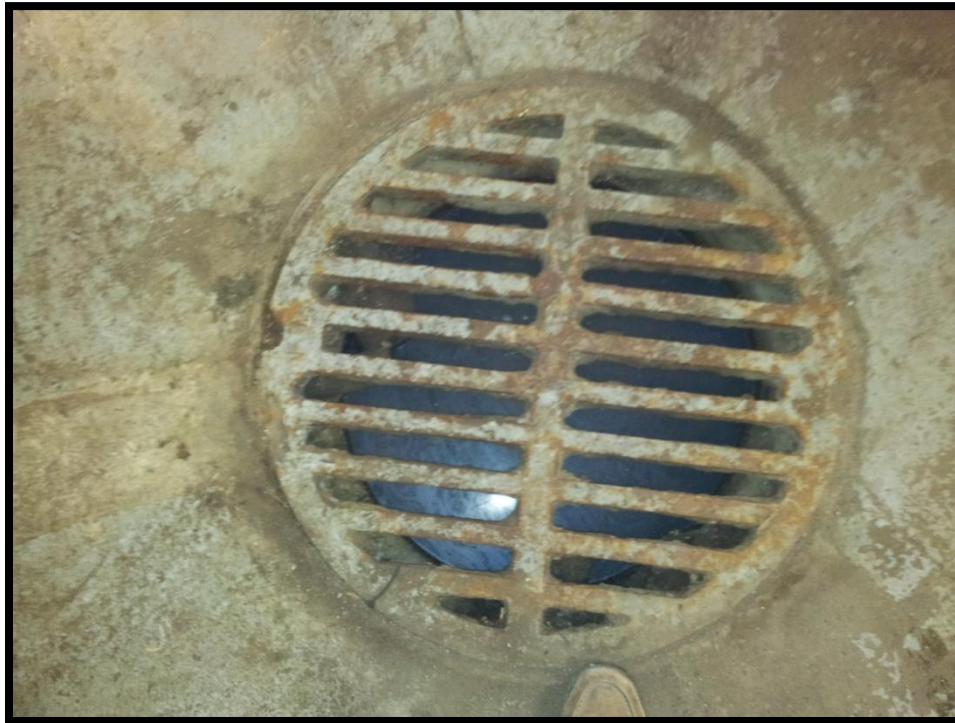
Photograph 3: View of drain in the landscaper's garage bay. Photograph depicts oil water with a film in the drain system.
