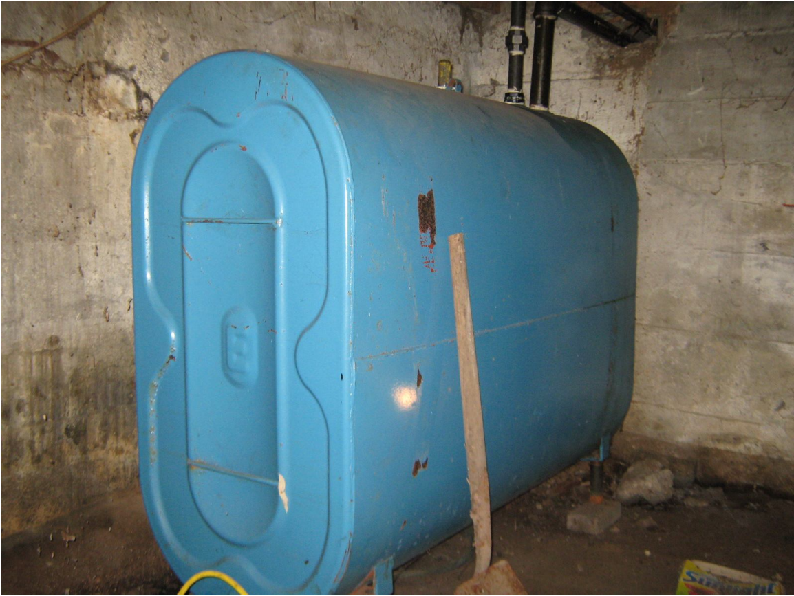
Photo 11: Furnace oil tank in basement crawlspace.
