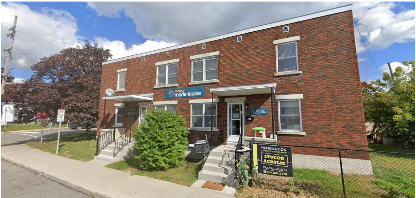
Figure 1: View of subject property at 233 and 235 Ste-Anne Avenue
