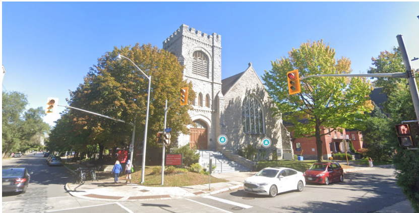
Figure 4 – View of the All Saints property
