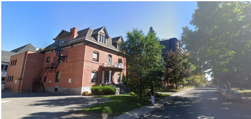
Figure 5 – View of 321 Chapel and existing office, with mid-rise residential in the background
