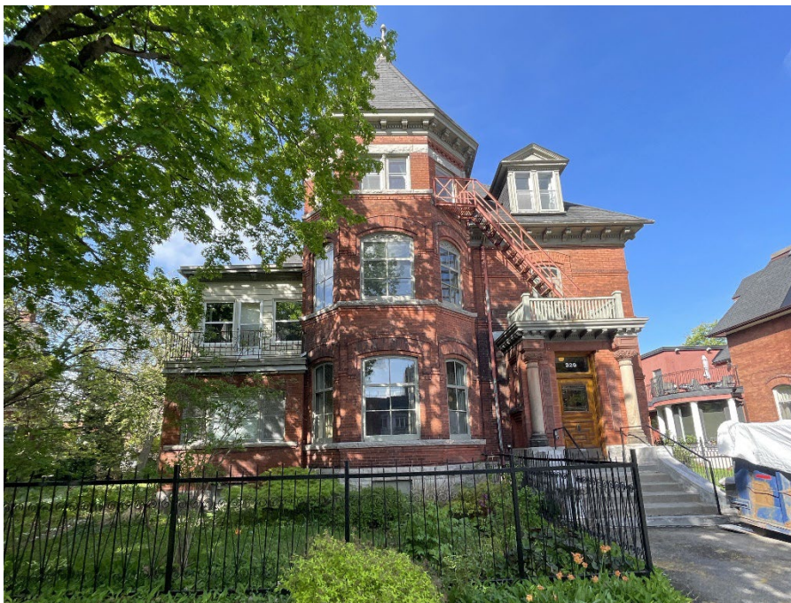
Photo 1 View of the east portion of Site Building A, May 20, 2026.
