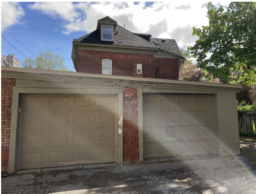
Photo 5 West view of Site Building B (foreground) and Site Building A (background), May 20, 2026.
