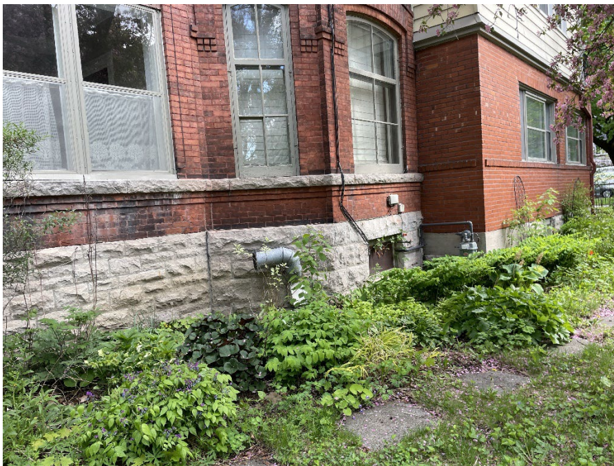
Photo 3 View of the southeast portion of Site Building A, May 20, 2026.
