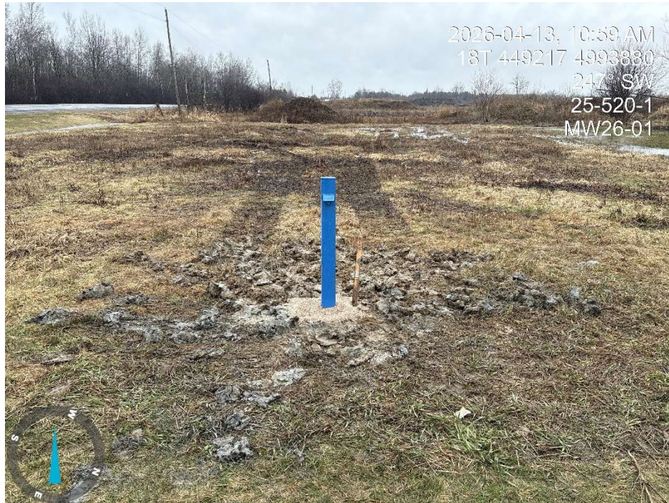
Photograph 1: Photograph of installed MW26-01.
