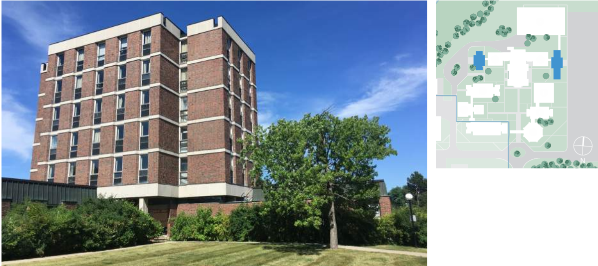
Figure 4. Building C, from novitiate courtyard (ERA, 2021).
