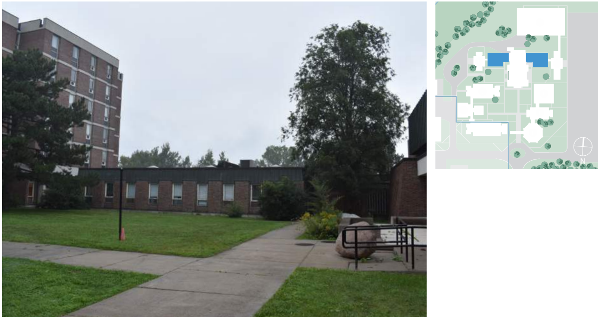
Figure 3. Building B, from Sisters' courtyard (ERA, 2021).
