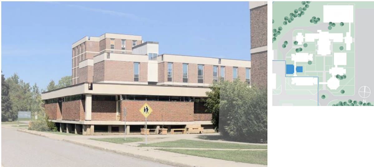
Figure 8. Building I viewed from southwest (ERA, 2021).
