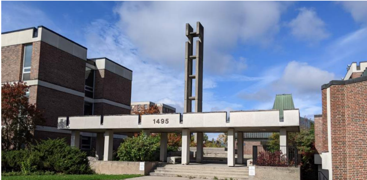
Figure 12. Main entrance canopy, with Campanile behind (ERA, 2021).
