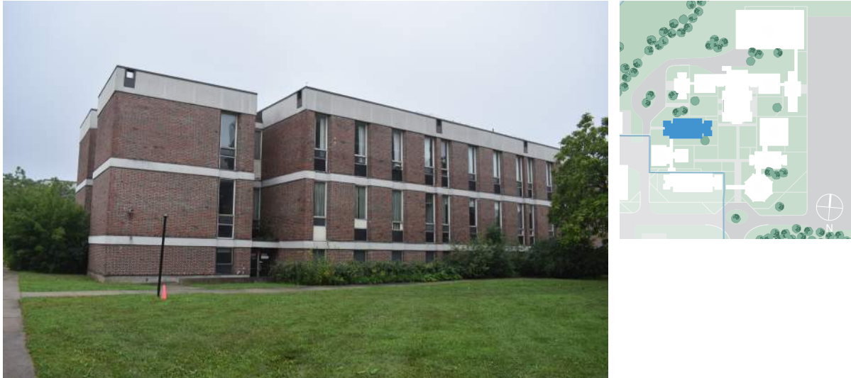
Figure 9. Building J, from Sisters' courtyard (ERA, 2021).
