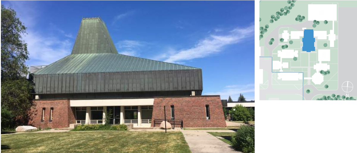
Figure 2. Building A, west elevation (ERA, 2021).
