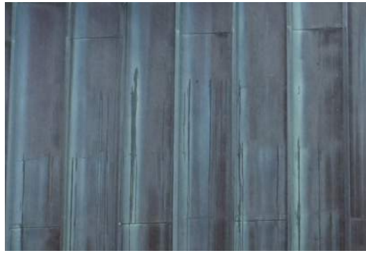
Figure 22. Standing seam copper roofing (ERA, 2021).
