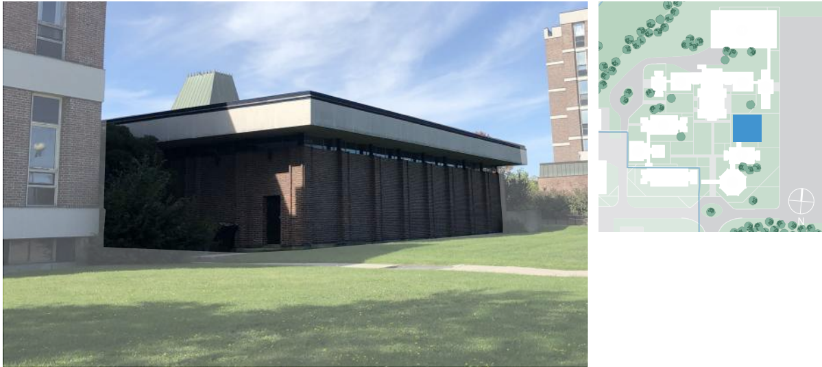
Figure 5. Building D, viewed from southeast (ERA, 2021).
