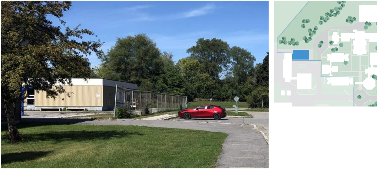
Figure 11. Building N, viewed from south-east (ERA, 2021).
