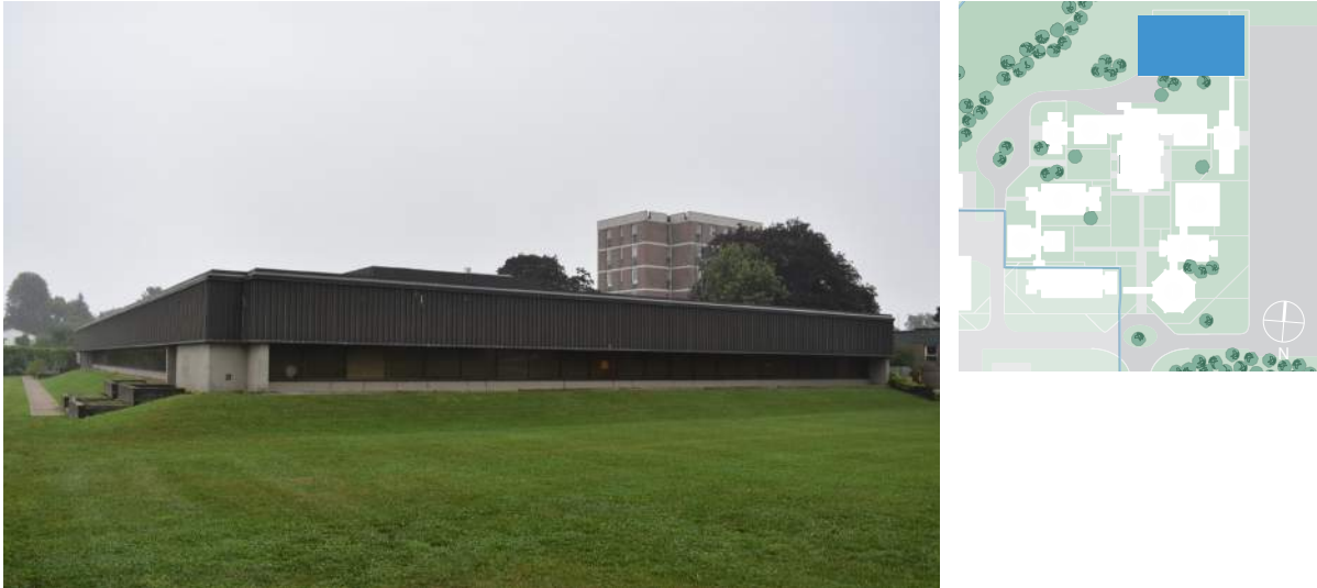
Figure 10. Building M, west elevation (ERA, 2021).
