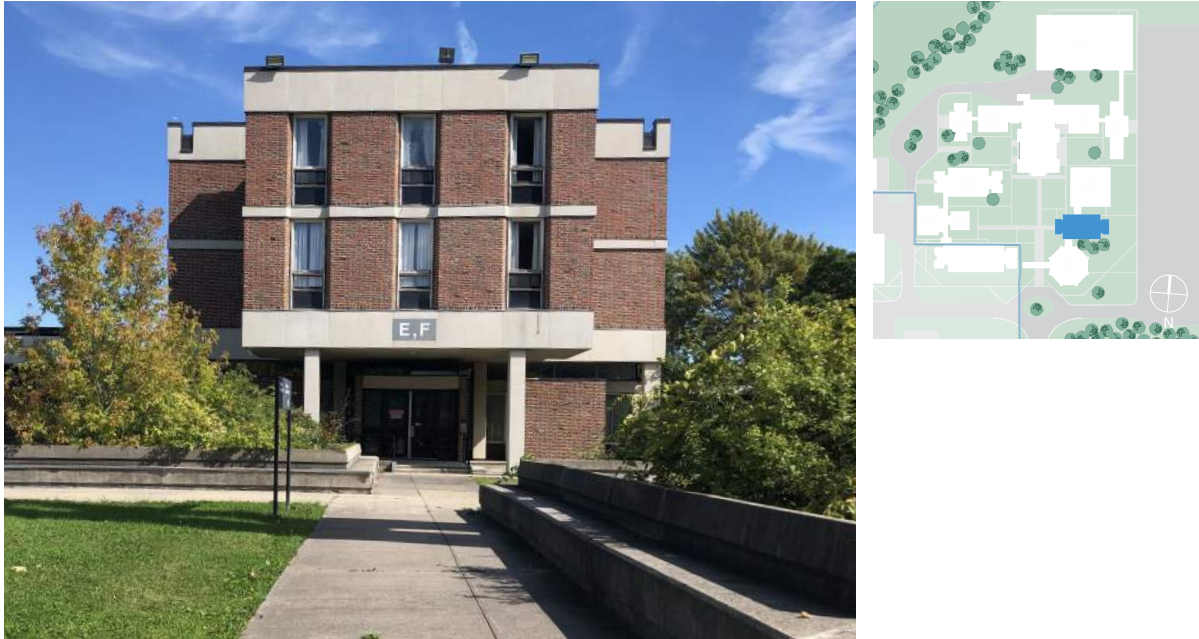
Figure 6. Building E, west elevation (ERA, 2021).
