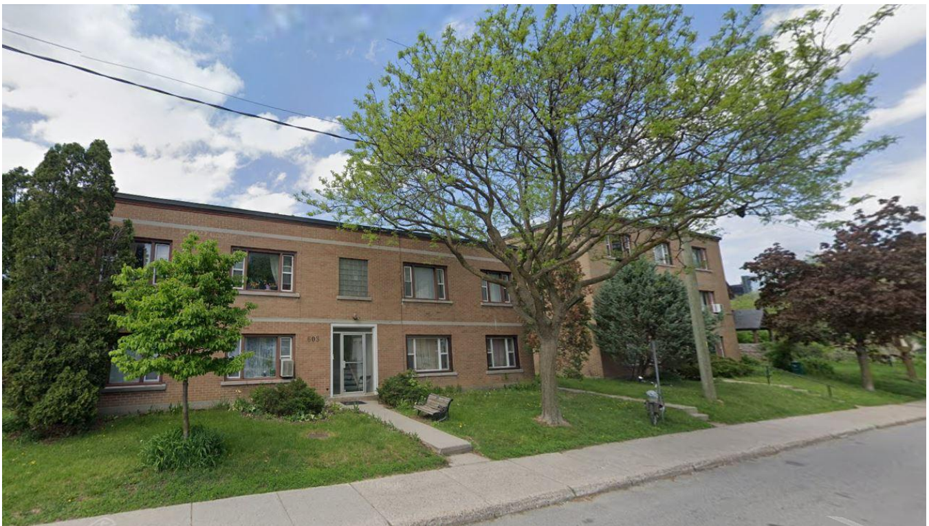
Figure 5 Streetview image of subject site looking northeast.
