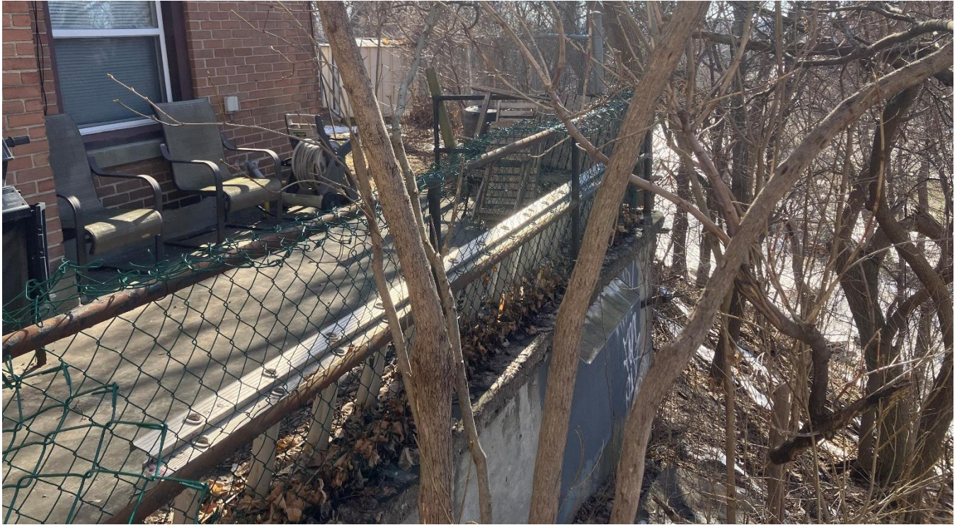
Figure 26 Escarpment existing condition.
