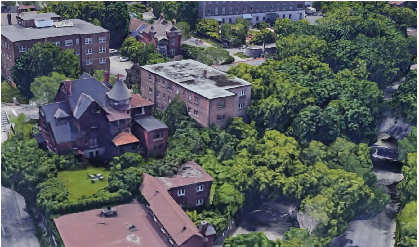
Figure 2: Aerial image of subject site looking southwest.
