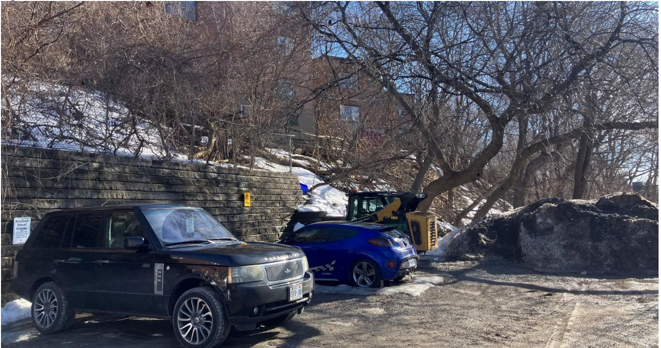
Figure 28 Escarpment existing condition.
