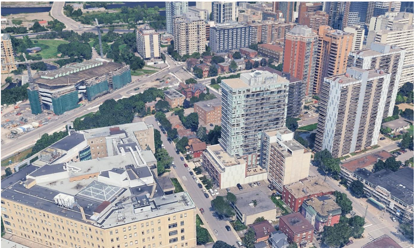
Figure 7 Aerial of site looking north.
