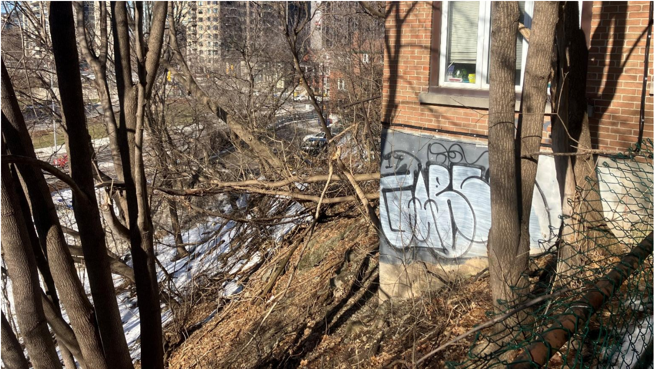
Figure 27 Escarpment existing condition.
