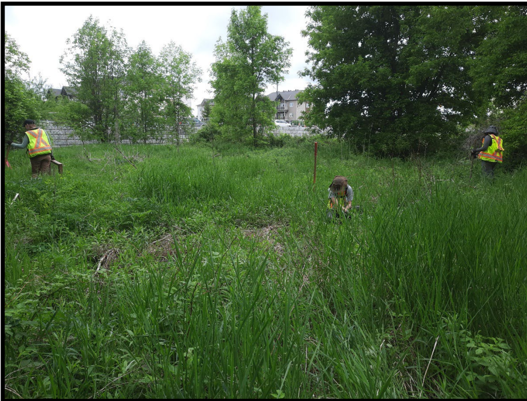
Figure 32: Test pitting in progress (MH1366-D221).
