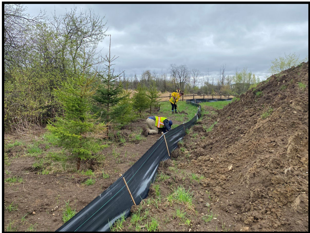
Figure 30: Test pitting in progress (MH1366-D077).
