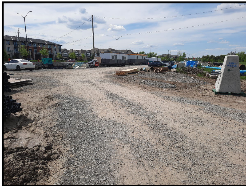
Figure 14: Staging area and work yard in southwest (MH1366-D192).
