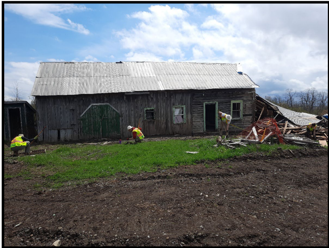
Figure 28: Test pitting in progress (MH1366-D031).
