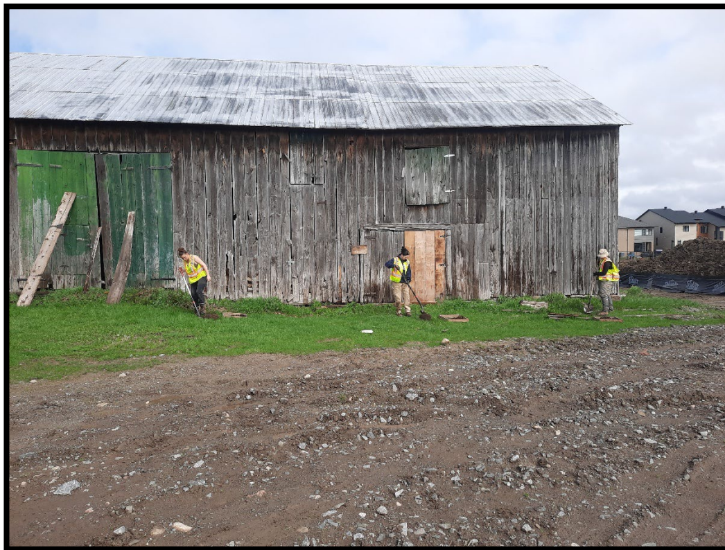
Figure 26: Test pitting in progress (MH1366-D009).
