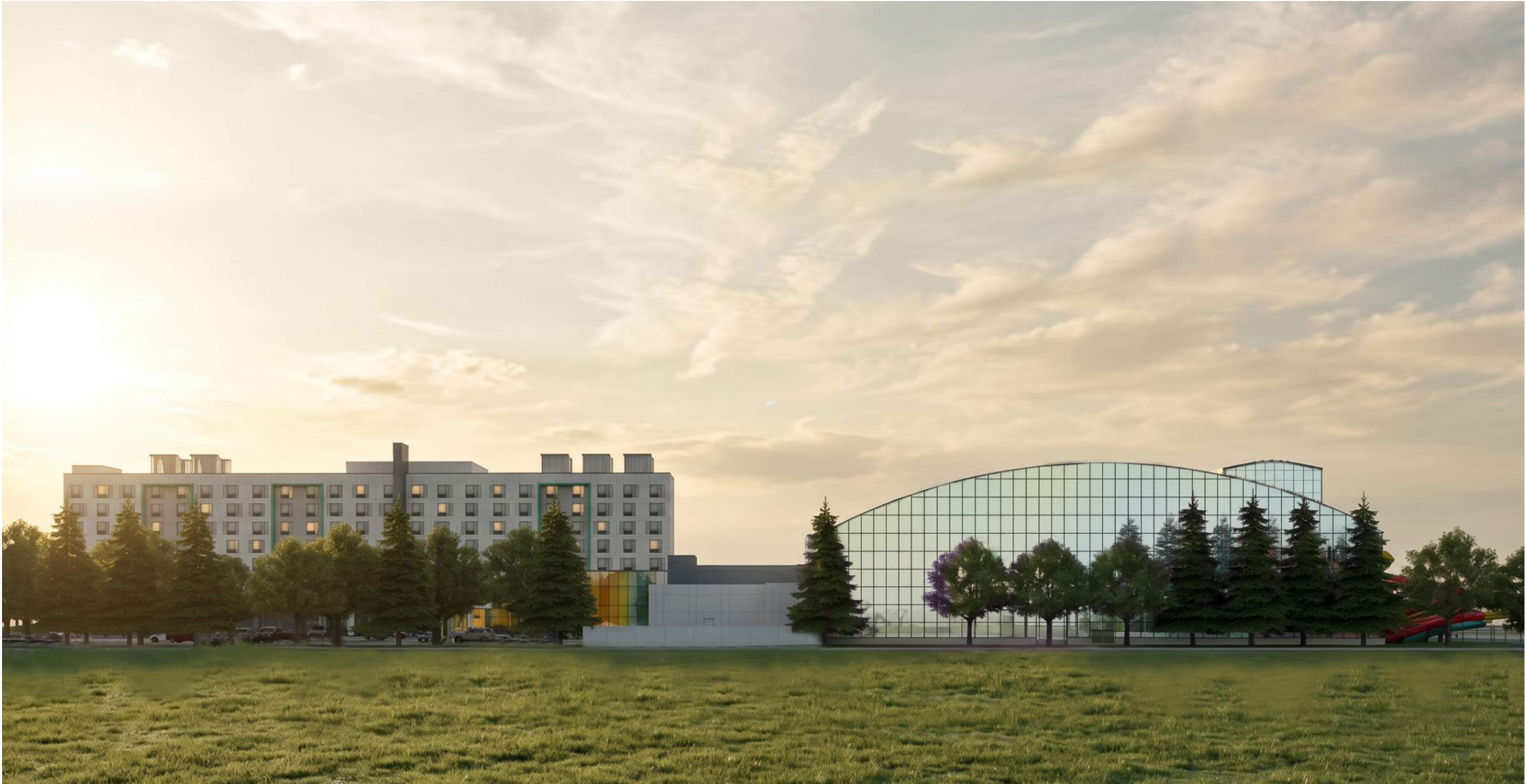
VIEW FROM DERREEN AVENUE
