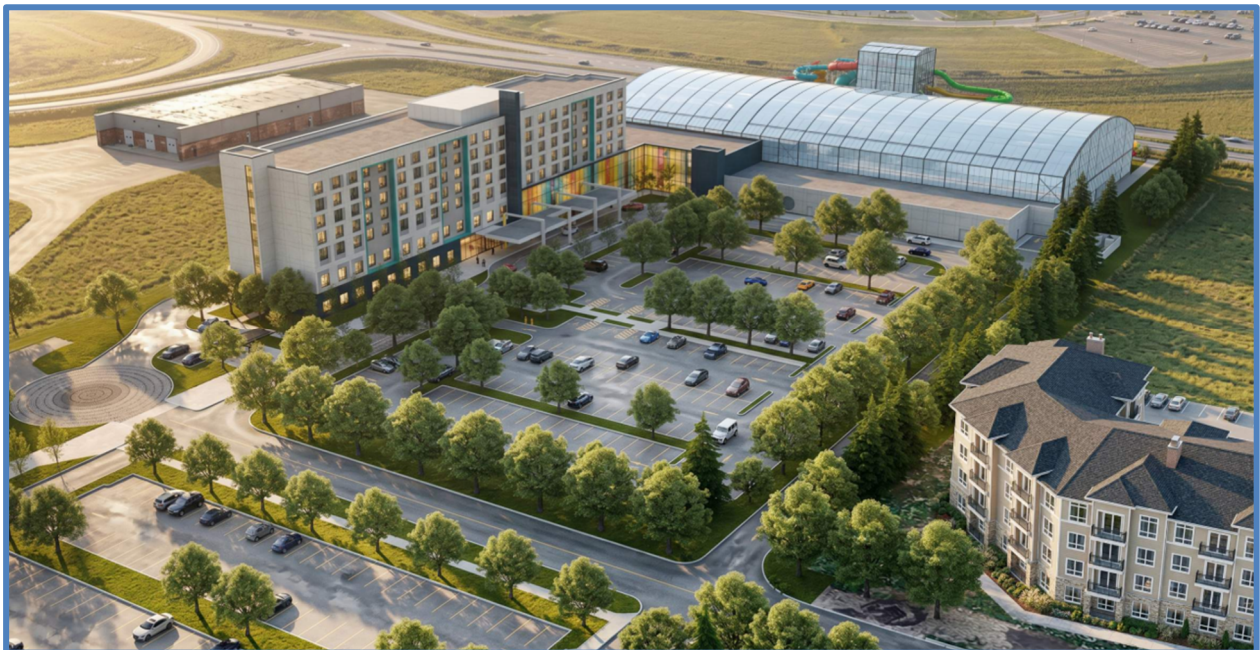
Figure 11: View of the Proposed Development Showing Culdaff Road
