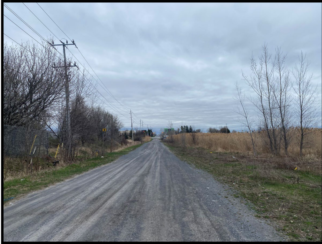
Figure 13: View along what will become Didsbury Road showing gas line buried utility (marked with yellow flags) along the southern side (MH1446-D050).
