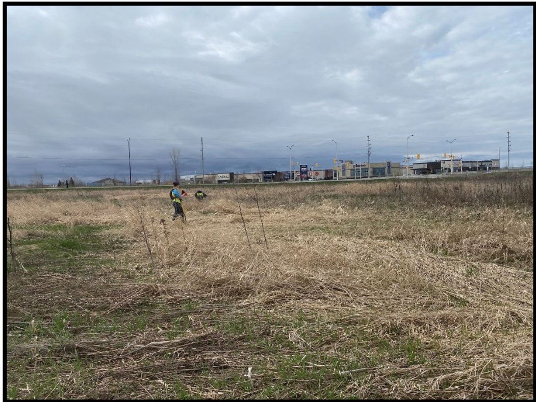
Figure 24: Test pitting in progress (MH1446-D067).
