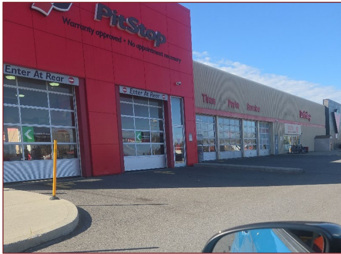
Photograph K5– Looking southwest at a vehicle service garage located southeast of the Site
