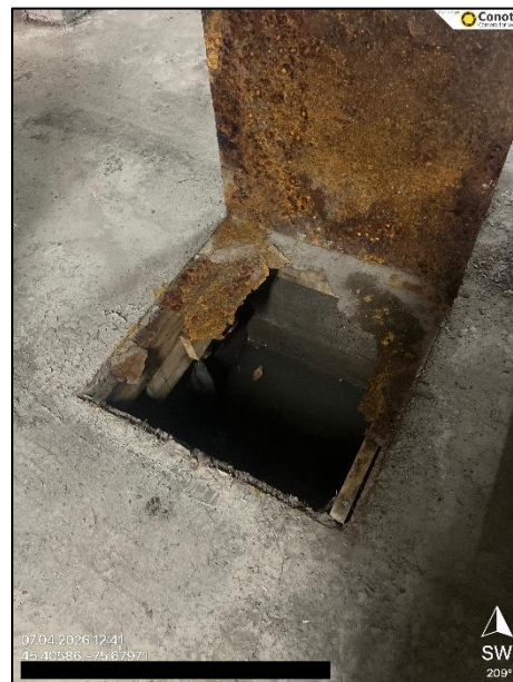
Sump observed in the mechanical room in the western portion of the on-site residential building
