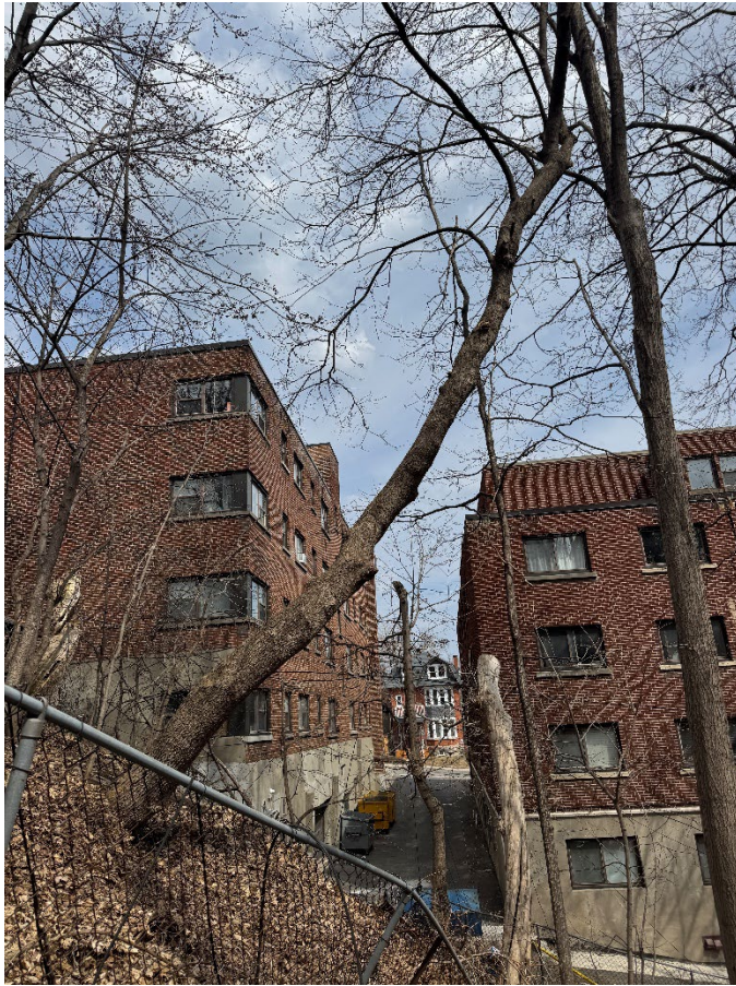
Photo 3: Tree 27, Manitoba maple on adjacent property that should be removed due to the potential for failure on subject property
