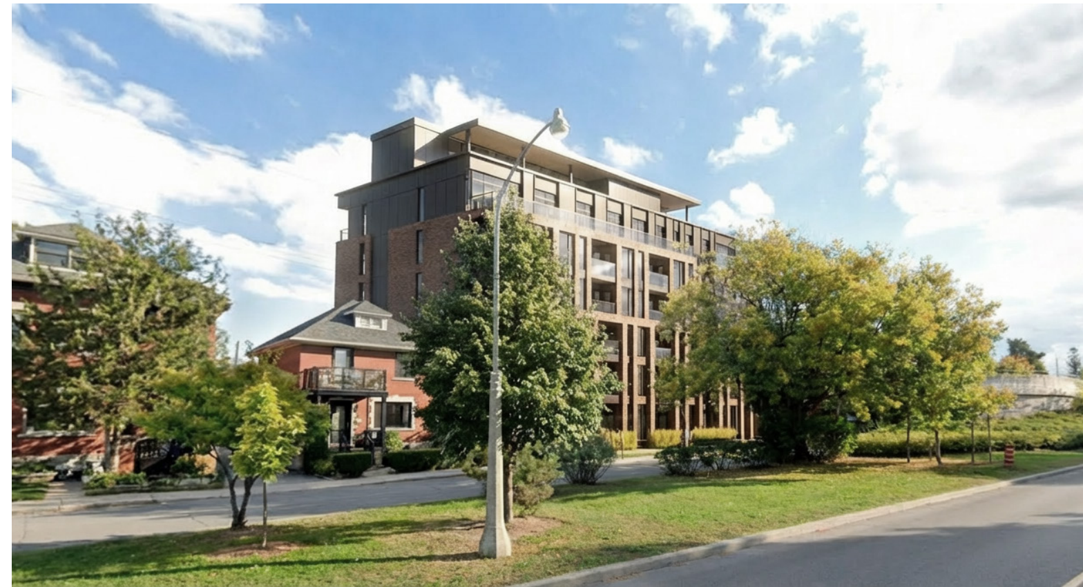
View From Colonel By Drive Looking South-East
