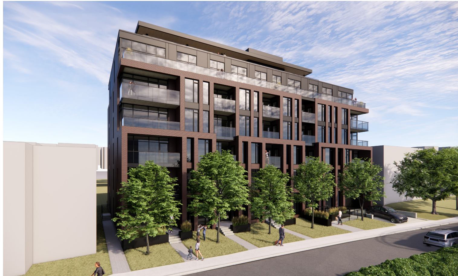
View of West Facade from Echo Drive
