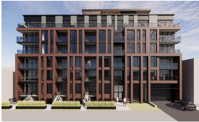
Original Design - West Facade
