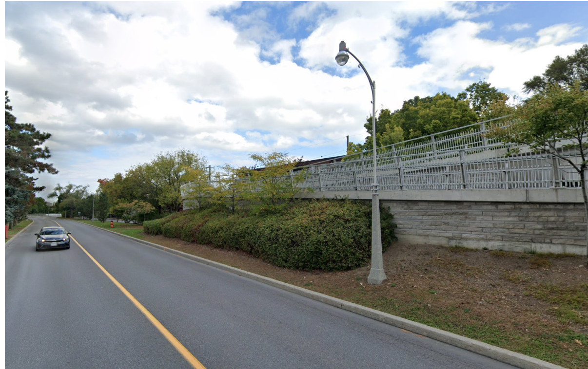
3. Looking North along Colonel By Drive
