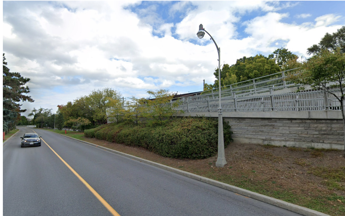
3. Looking North along Colonel By Drive
