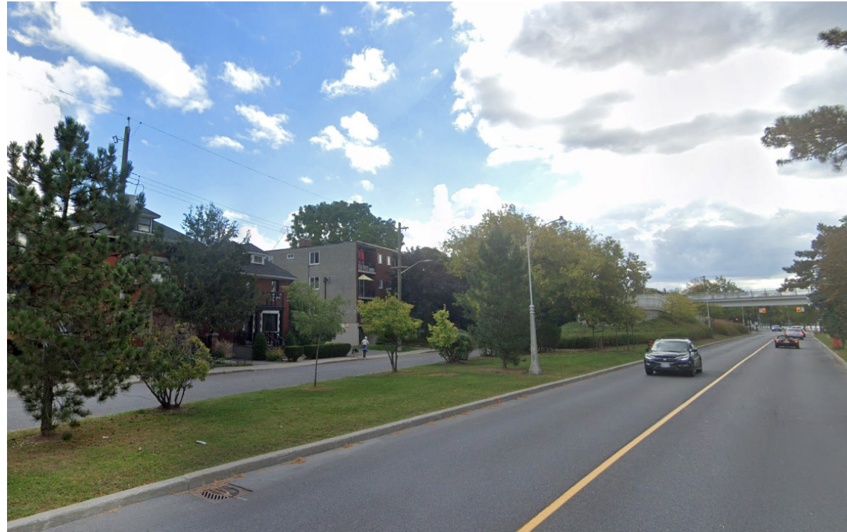
1. Looking South along Colonel By Drive
