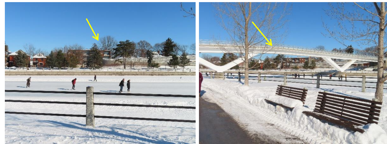
Figure 9: Views of the existing property obscured by the Flora Footbridge, photographed from the West side of the Canal (Source: Juxta Architects).
