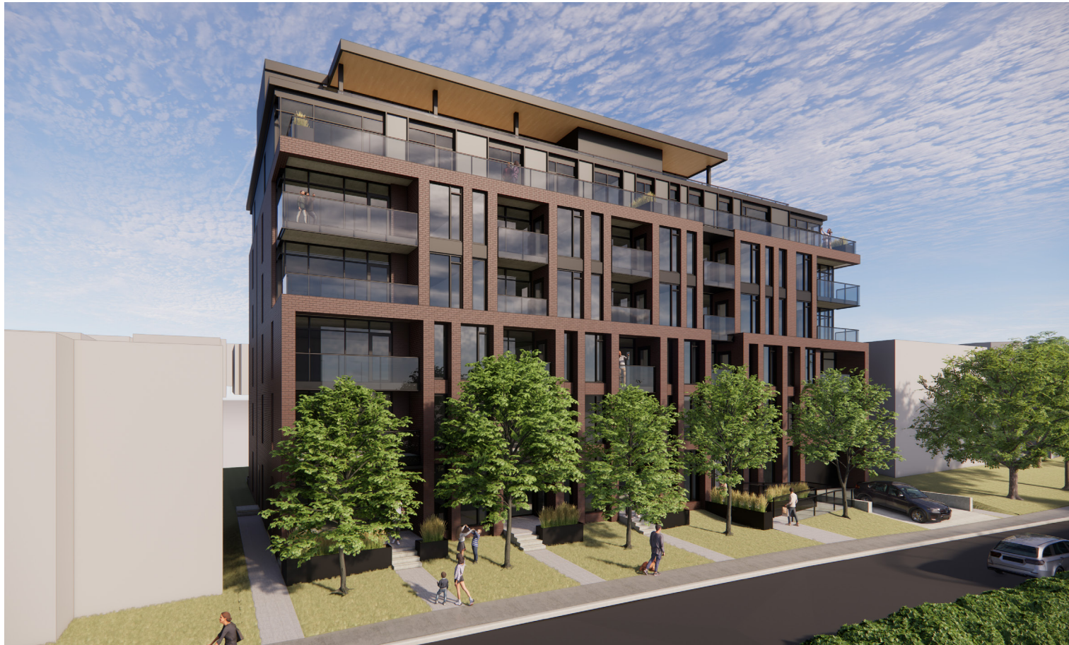
View of West Facade from Echo Drive
