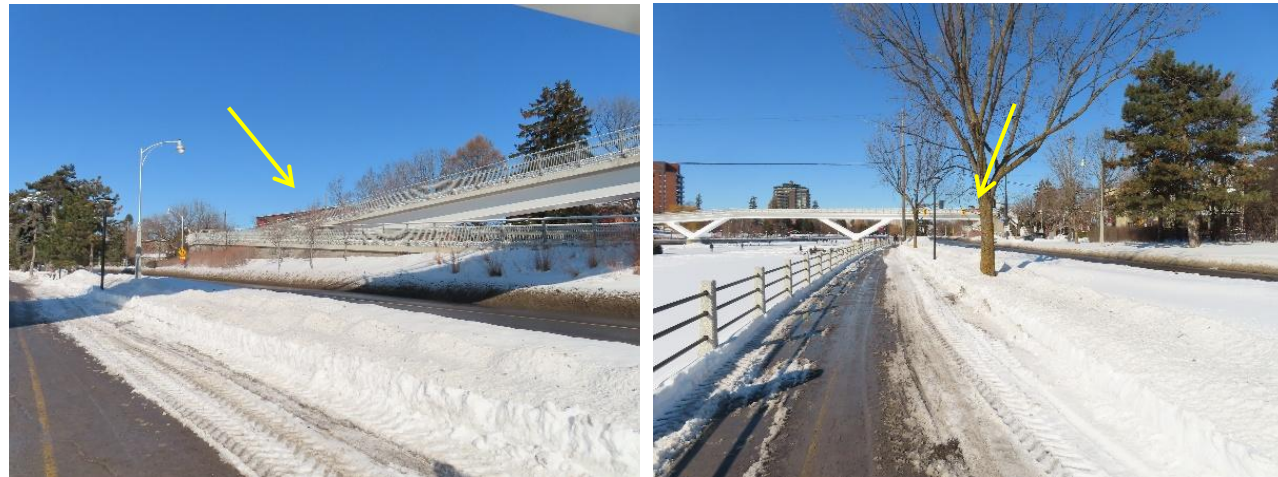
Figure 8: Views of the existing property obscured by the Flora Footbridge, photographed from the East side of the Canal (Source: Juxta Architects)
