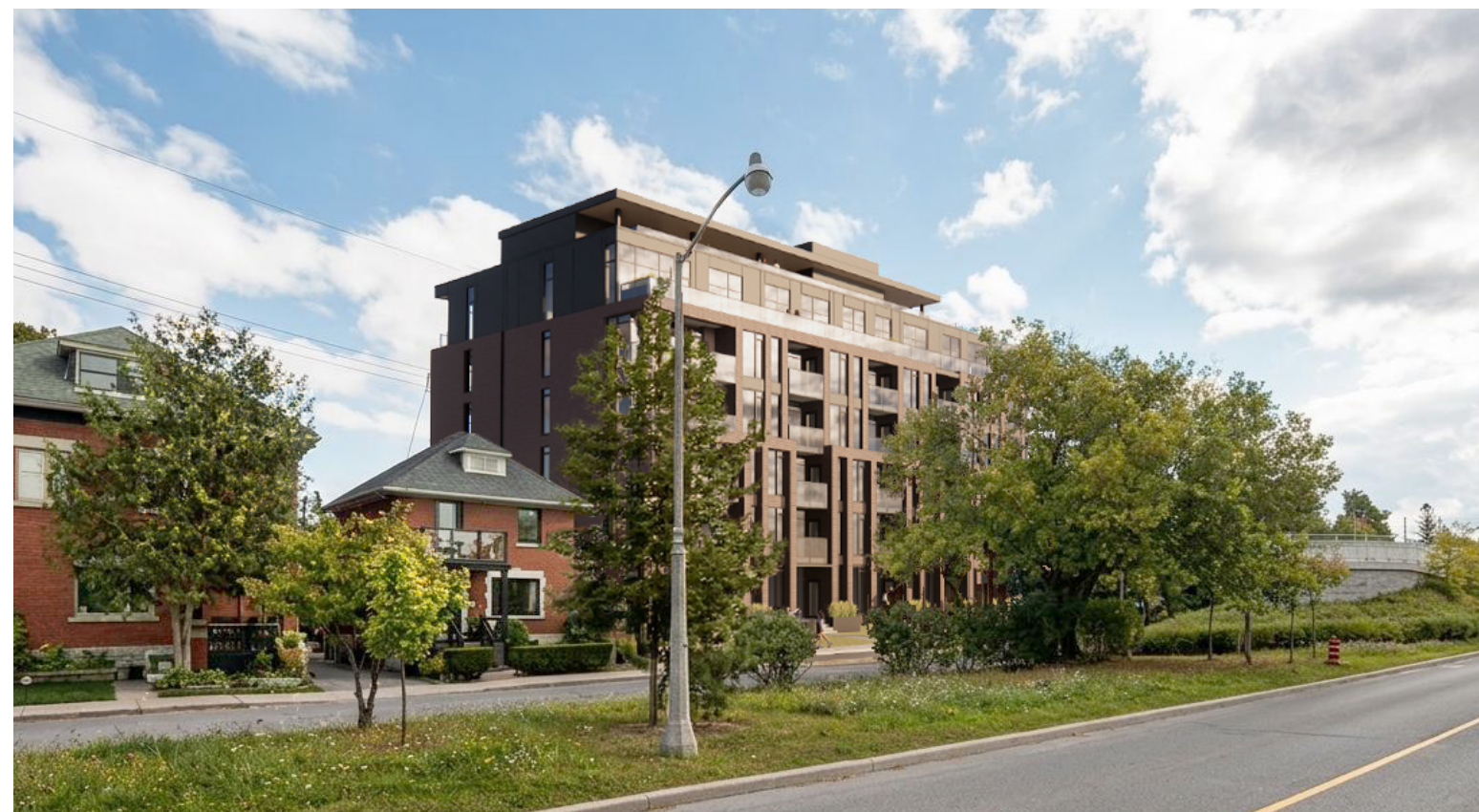
View From Colonel By Drive Looking South-East
