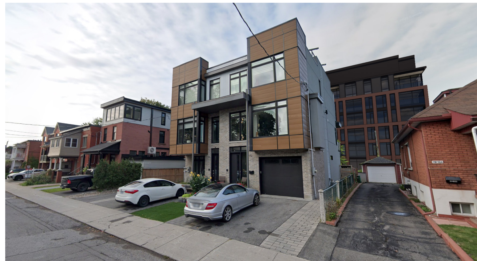
View From Colonel By Drive Looking South-East
