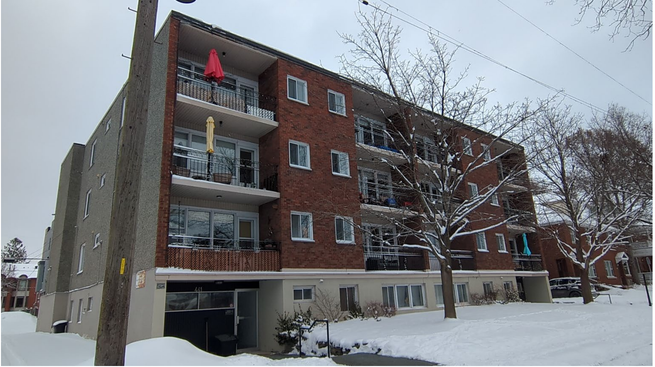
Figure 2: Subject site looking southeast from Echo Drive.
