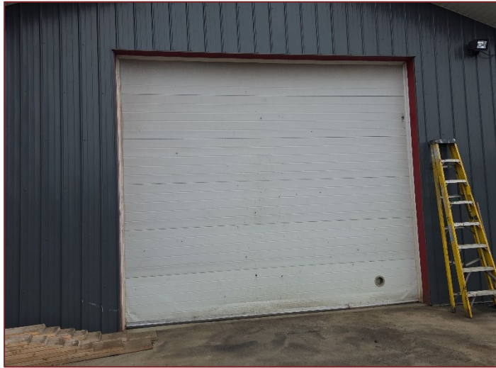
Photograph K5 – Looking east at the entrance of the large shop.
