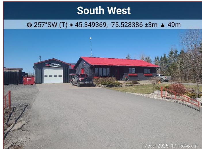
Site Photograph 2: CVC_1 – Commercial – Business Sector
