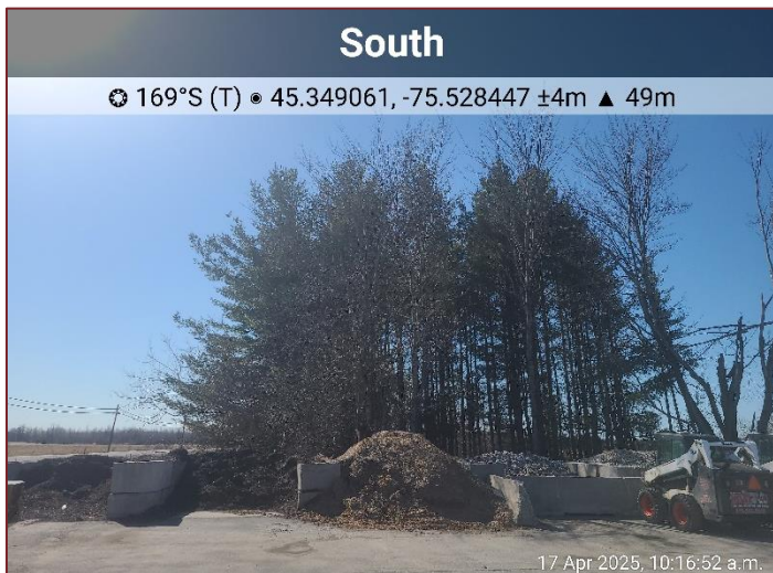
Site Photograph 3: CVC_1 – Commercial – Business Sector
