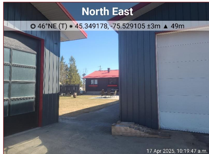
Site Photograph 8: CVC_1 – Commercial – Business Sector
