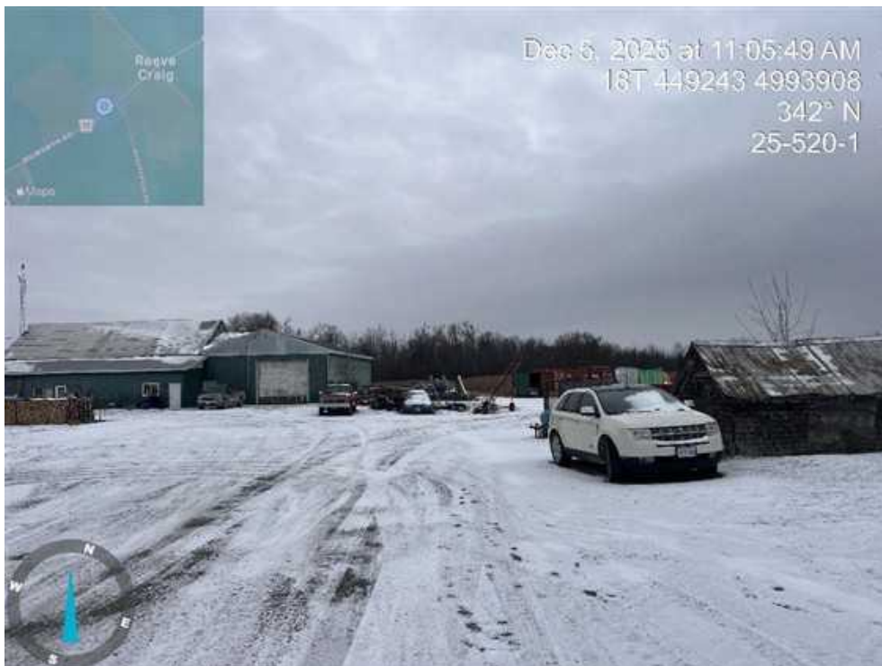
Photograph 4 – View of the commercial service garage.
