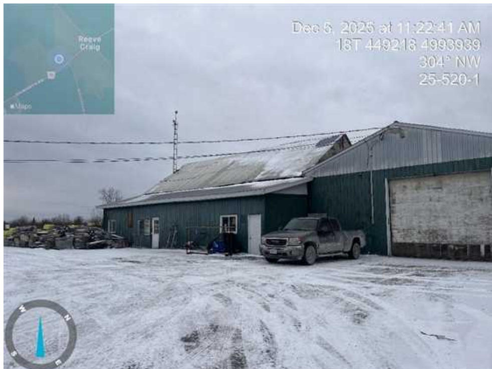
Photograph 16 – View of the commercial service garage.
