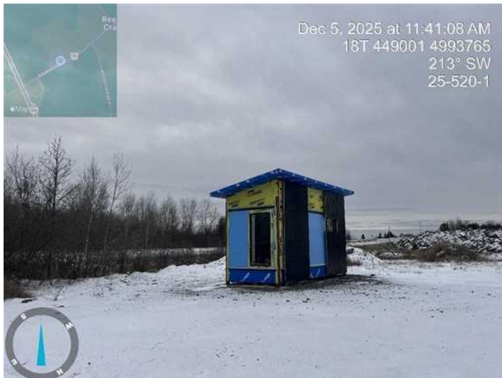
Photograph 20 – New structure located on the southern elevation of the Site, just off of Dilworth Road.
