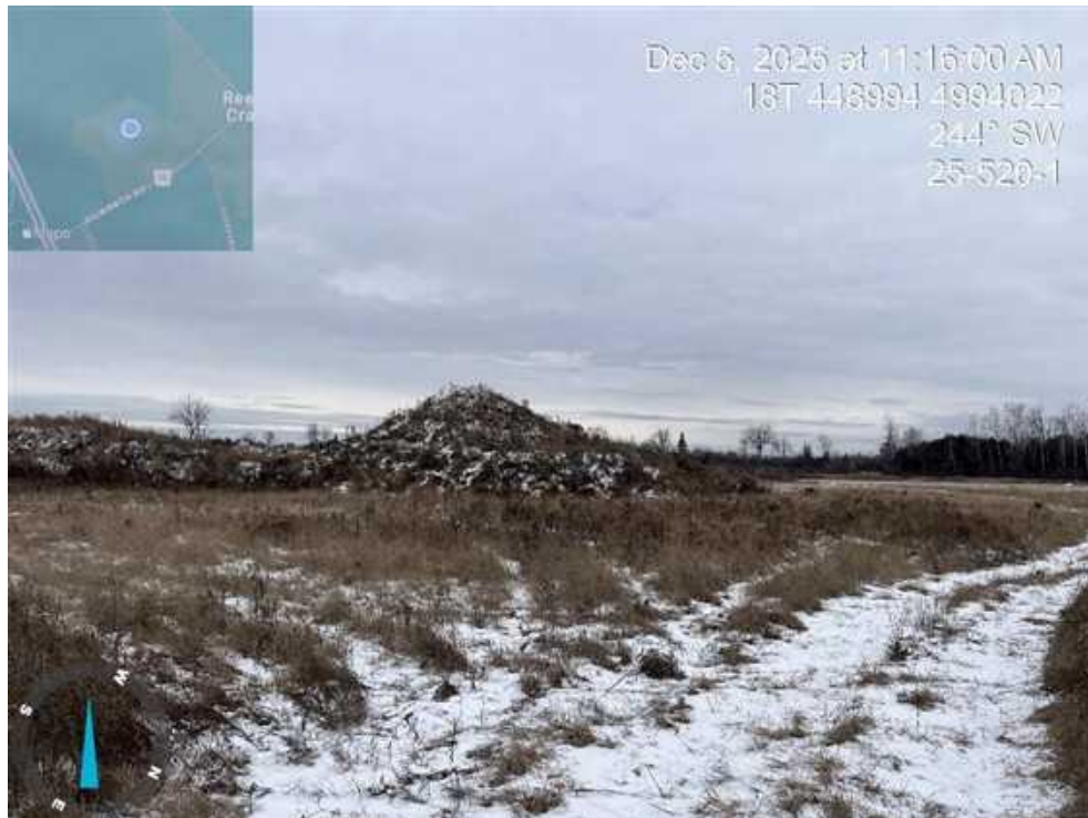
Photograph 15 – View of the central/northern portion of the Site.
