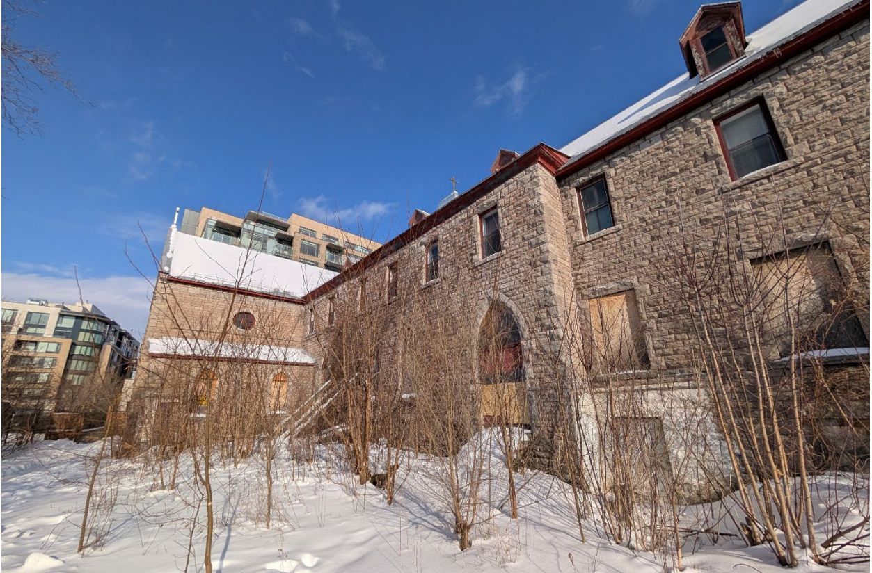
Figure 8: West elevation of convent wing and chapel at northwest corner of the complex. (Heritage Studio, January 2026)
