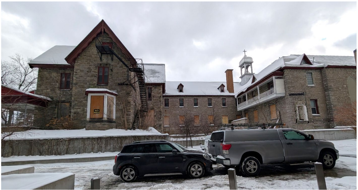
Figure 6: North elevation of Gothic Revival house, north wing and chapel. (Heritage Studio, January 2026)
