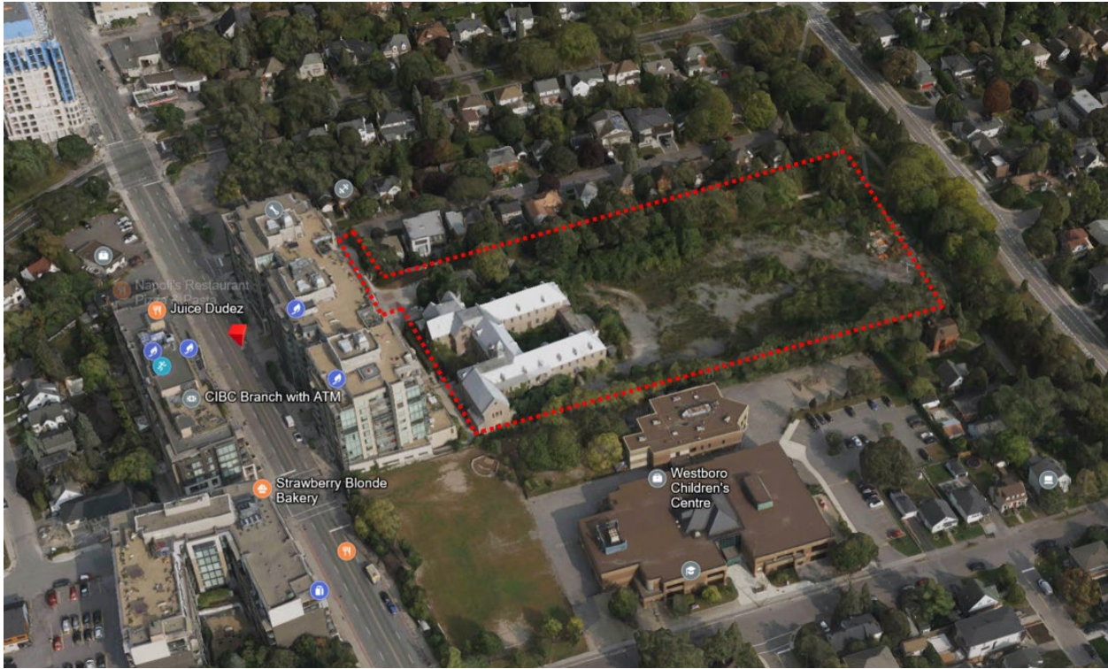
Figure 1: Bird's eye aerial photograph of the subject property. (Bing Maps, annotated by Heritage Studio).
