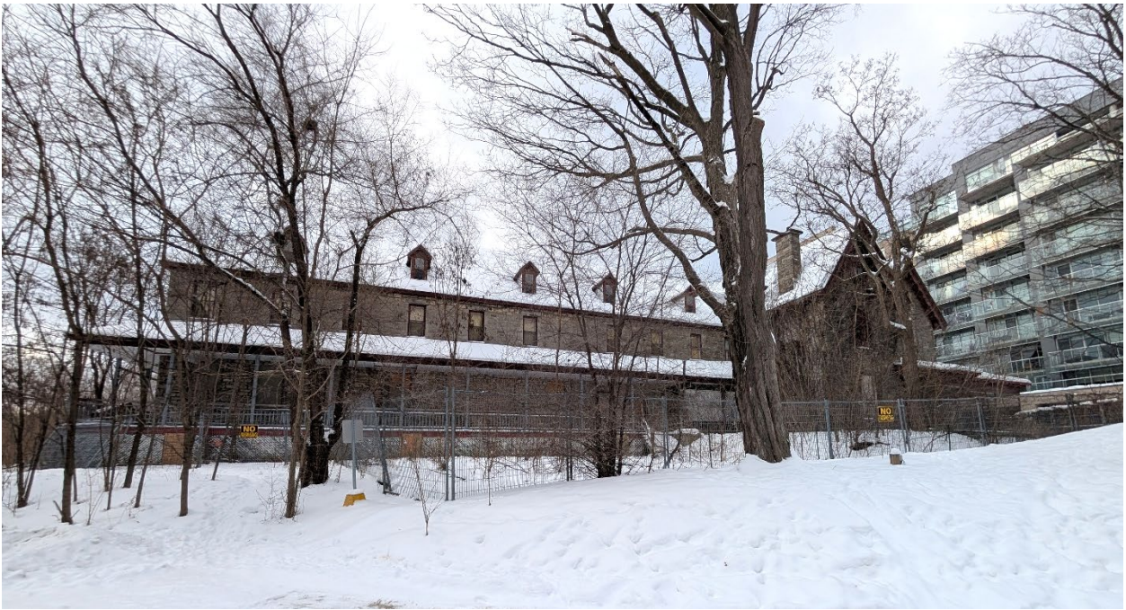
Figure 7: East elevation of the east wing and Gothic Revival house. (Heritage Studio, January 2026)
