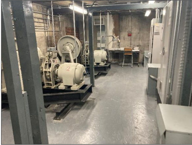
Photo 5 – Interior photo of the elevator maintenance room.
