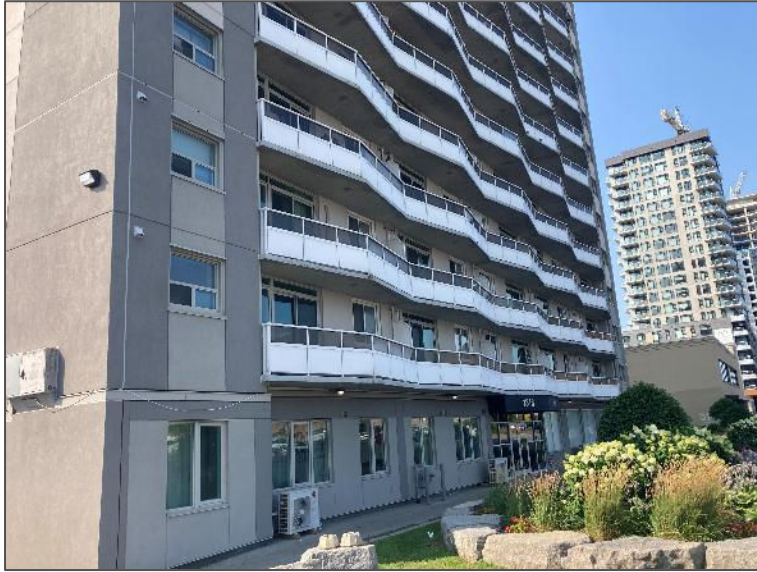
Photo 1 – Northwest elevation of the Site Building, looking southeast.
