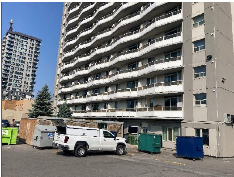
Photo 4 – Southeast elevation of the Site Building, looking northwest.
