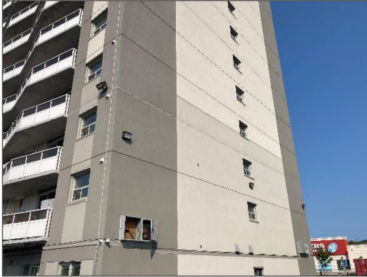
Photo 3 – Northeast elevation of the Site Building, looking northwest.
