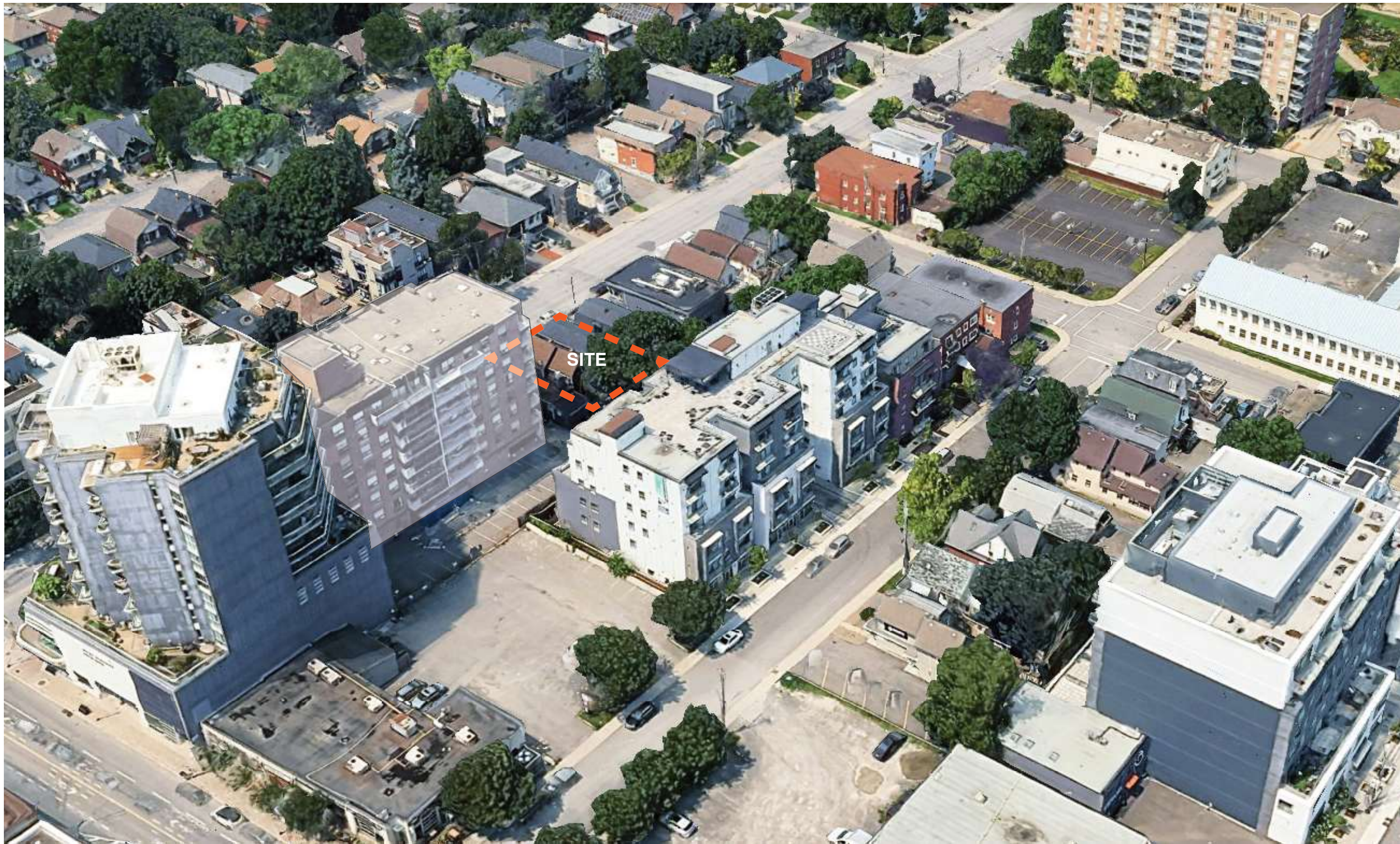
.10 AERIAL VIEW FROM NORTH EAST
