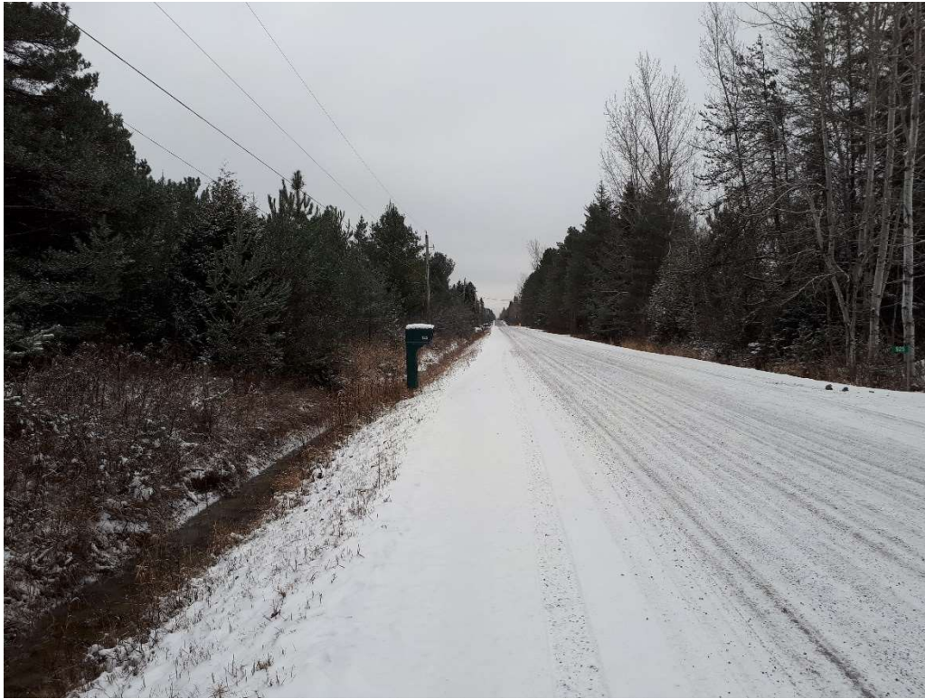
Photograph 3: David Manchester Road, looking south. Phase I Property on the left.
