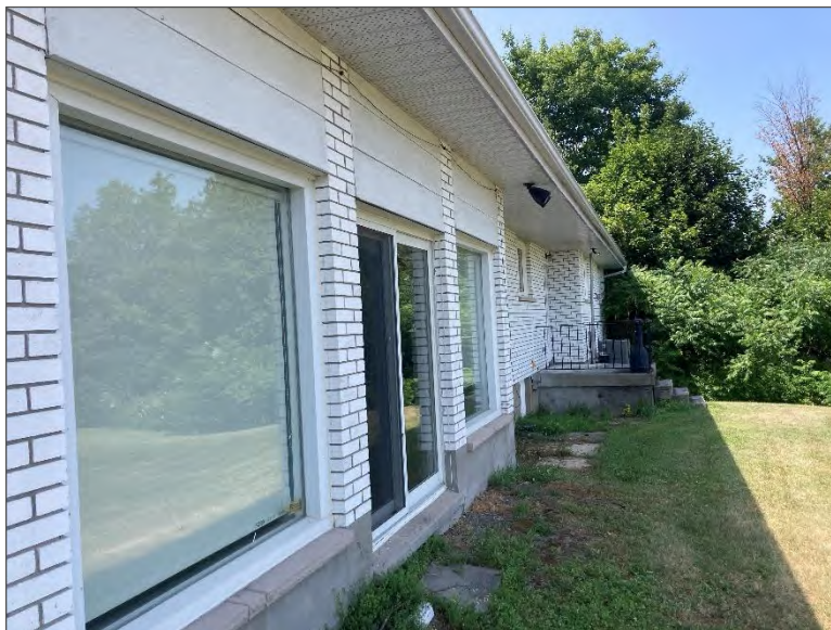
Photo 2 – Site Building B (northeast elevation).
