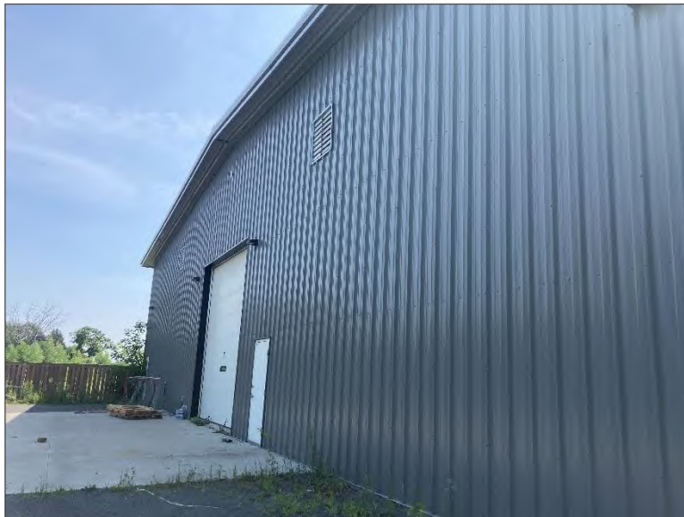
Photo 4 – Site Building A (southwest elevation).
