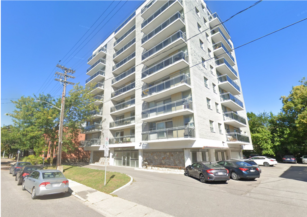
Figure 4: Directly across the street from the subject site on Nelson Street.
