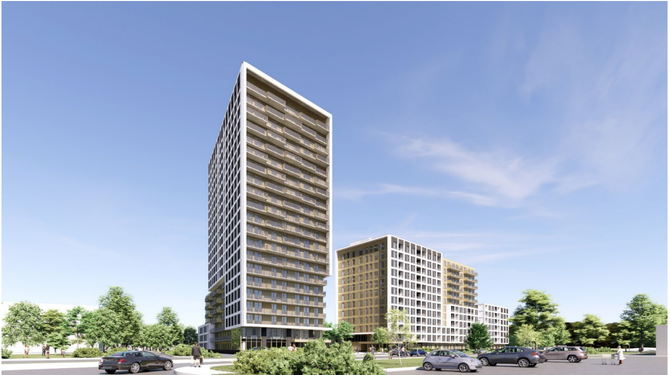
Figure 9. View looking southwest towards Hazeldean Road
