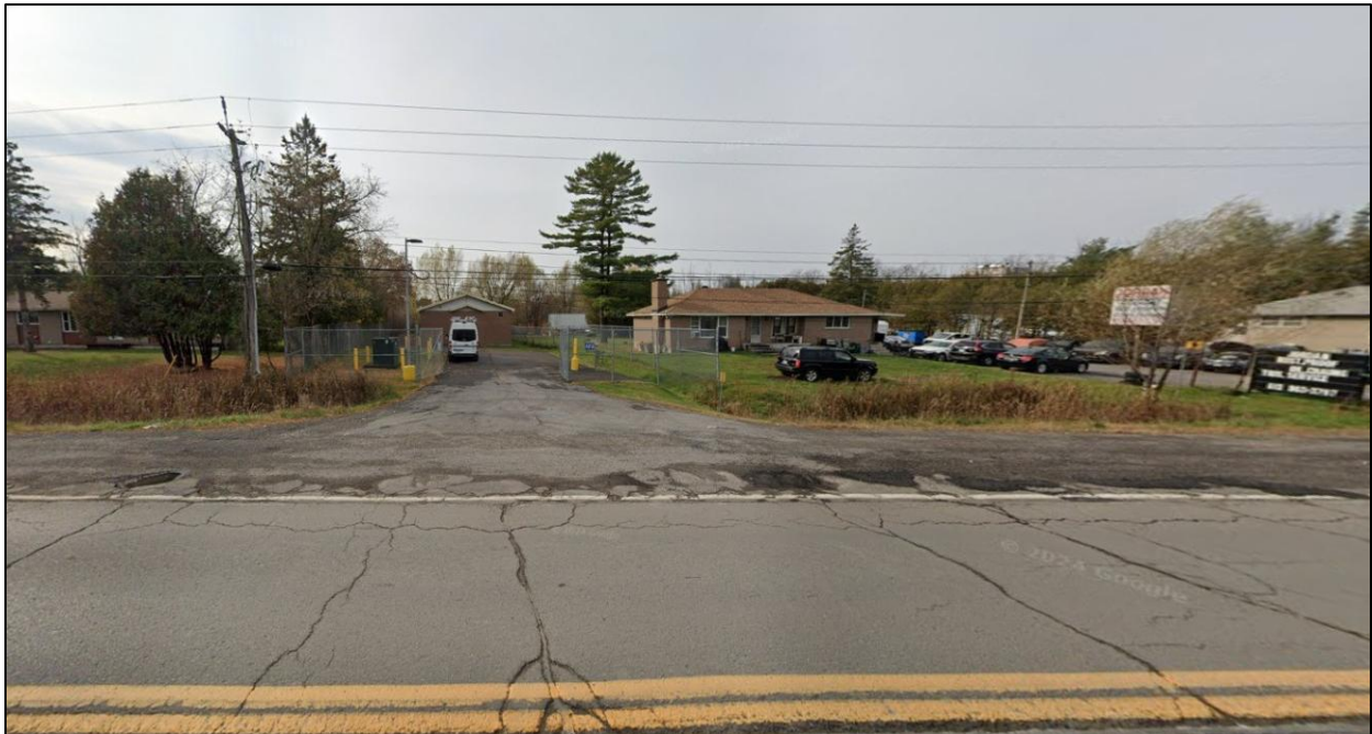
Figure 3: Existing automobile service station and dealership as well as the municipal water pumping station are located east of the Subject Site looking west from Bank Street (Google Streetview 2024).
