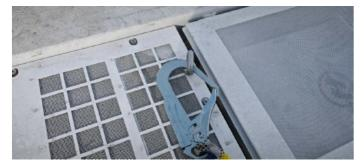
figure 5-34 Schematic Diagram of Connecting Safety Buckle
