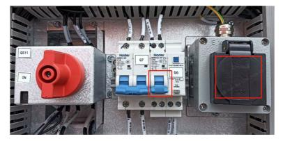
**Step 16** Turn on the filling-draining kit switch. The pump working indicator of the filling-draining kit will come on, and the pump starts to fill coolant.
