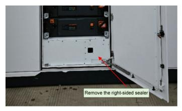
figure 5-28 Right Sealing Plate
