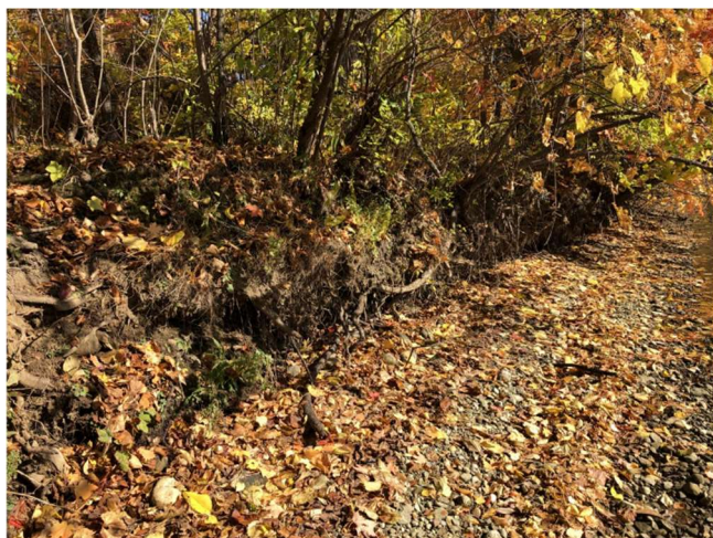
Photo 1: View looking upstream at S1 on October 14, 2022.
