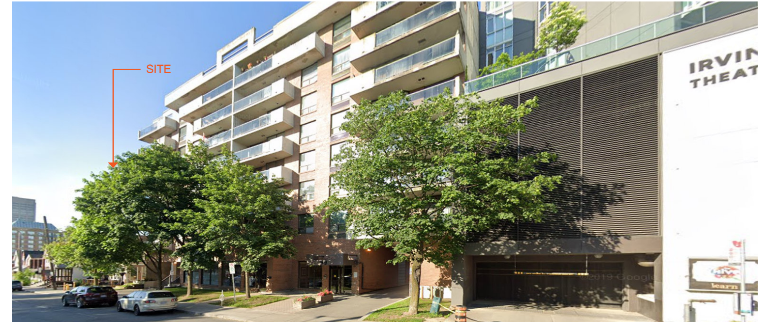
2 - VIEW FROM HOLLAND LOOKING NORTH
