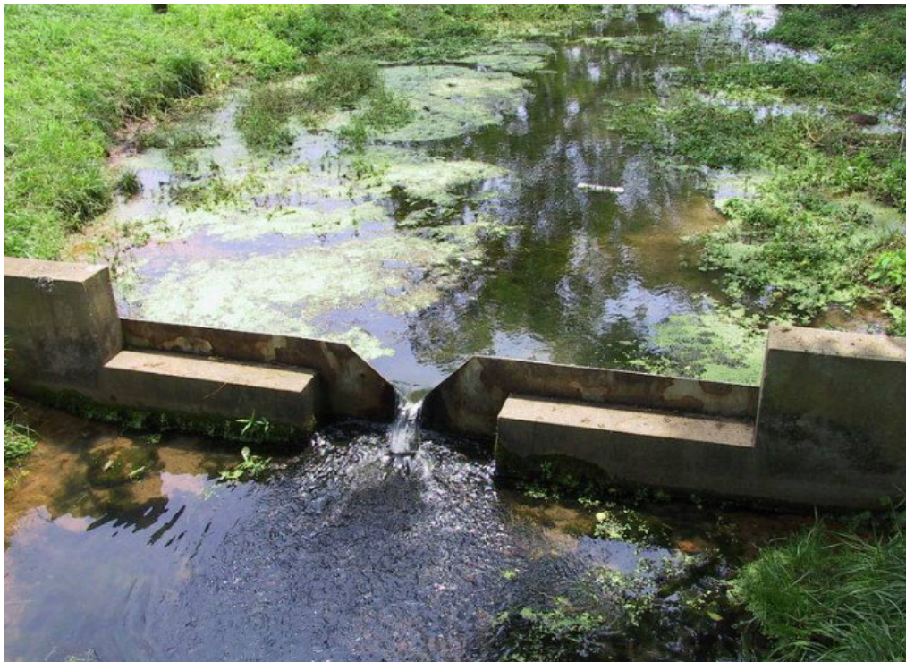
Figure 6-1: V-notch Cast-In-place Concrete Weir Wall Illustration
