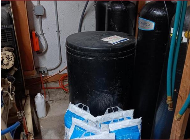
Photograph L5 – Boiler used on site property. Stored within barn.
