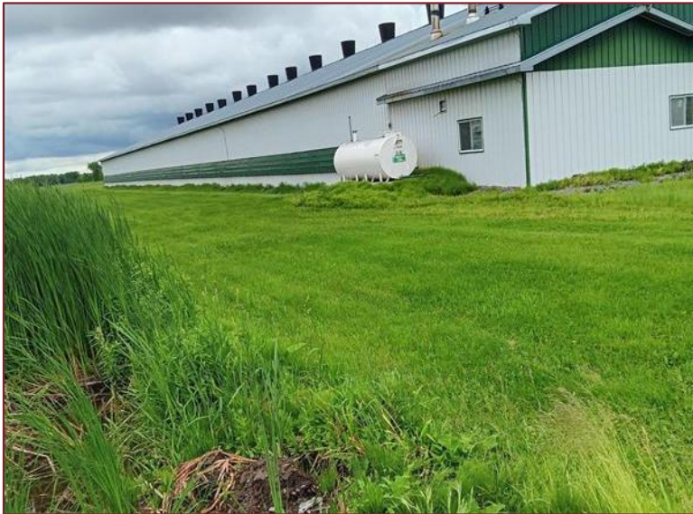
Photograph L15 – Looking south at the adjacent barn’s furnace oil tank. Parcels of land are separated by a small ditch.
