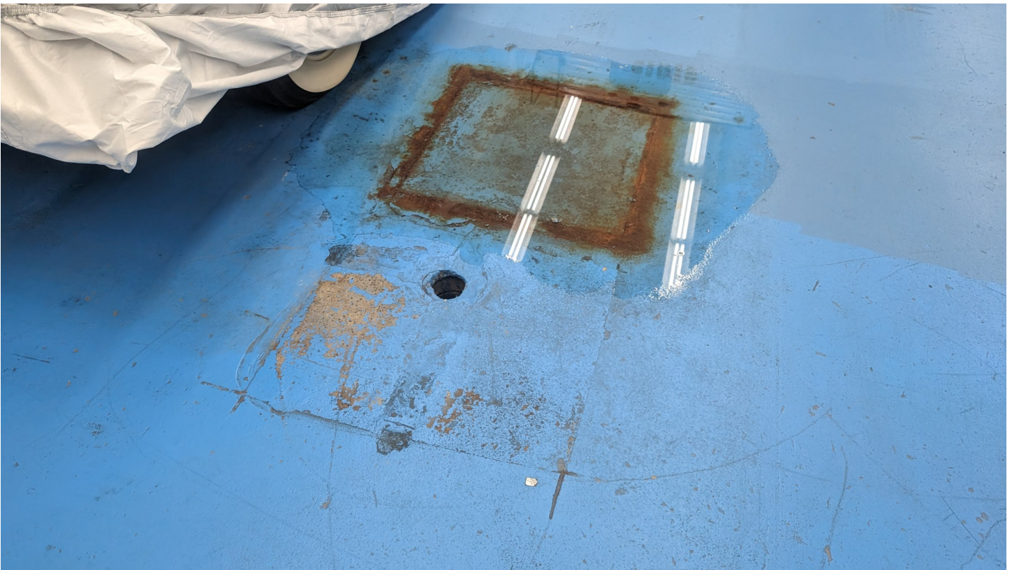
Photo K8 - A cut out (potential location of the former oil water separator ) was noted in the floor of the building.
