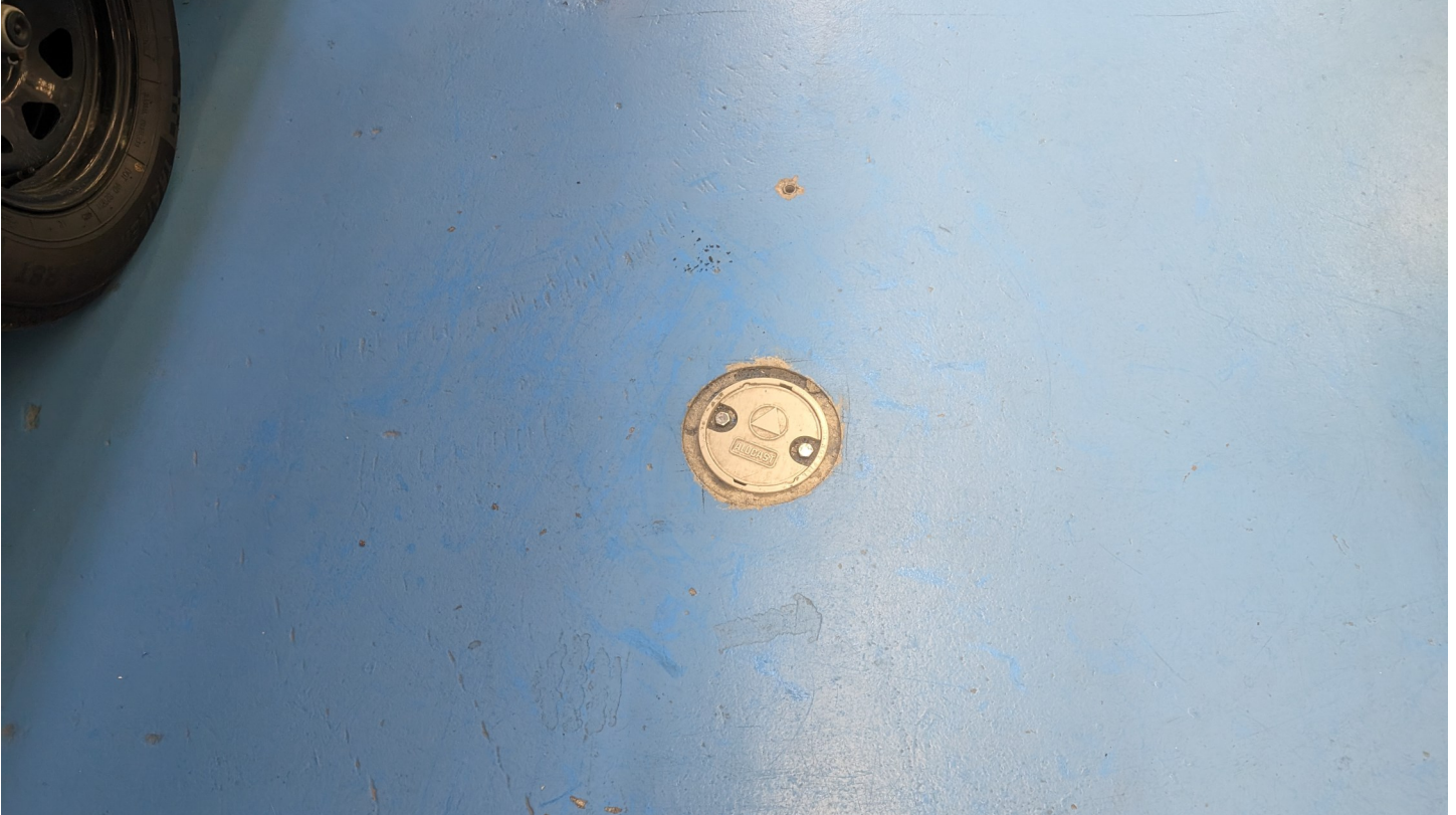
Photo K7 - Monitoring well was located inside the on-Site structure. The concrete floor was in a good condition with minimal cracking.
