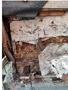
Figures 5 and 6 : The two views illustrate the multiple layers of finishes covering the squared timber, (tin panels insul-brick, ridged insulation, and vinyl siding.) Source David Yoo 2022.
