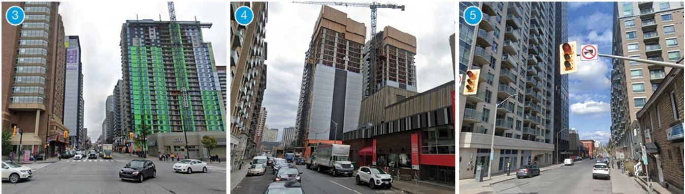
Figure 2: Street views of the subject property from varying locations.
