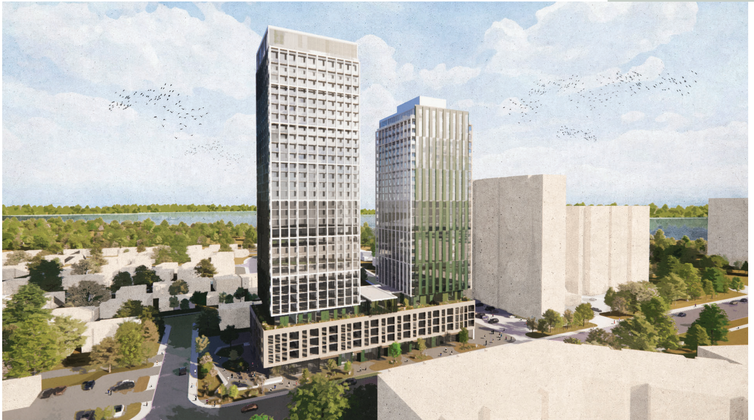
View of the Site Looking North
