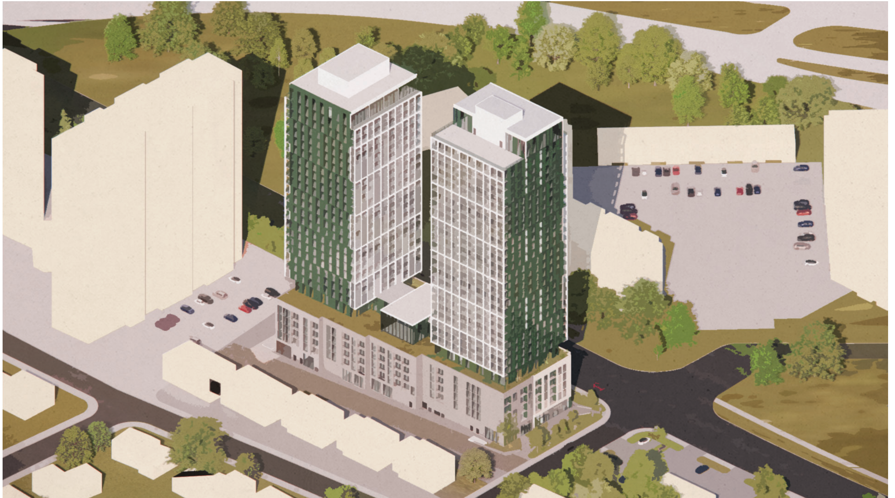
Aerial View of the Site Looking South
