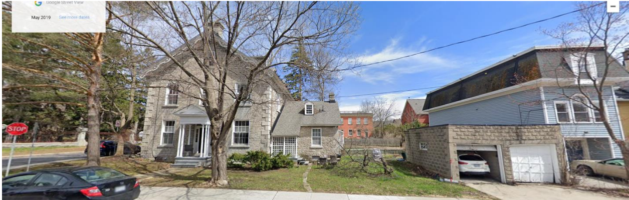
Figure 5: Elevation at 71 Thomas Street with the Boyd block 2-car garage. The red brick building in the background is the Vietnamese Embassy Source: Google Maps 2024.
