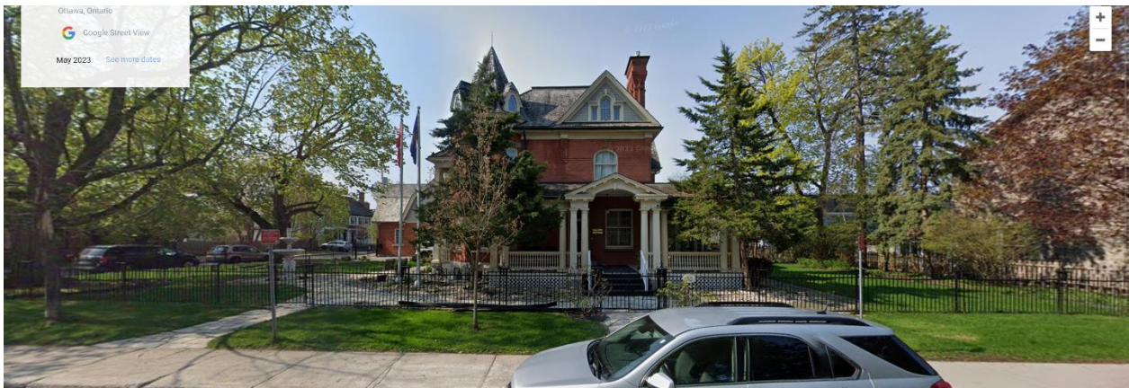
Figure 9: A view of 55 MacKay Street, the Vietnamese Embassy. Source Google Maps 2024
