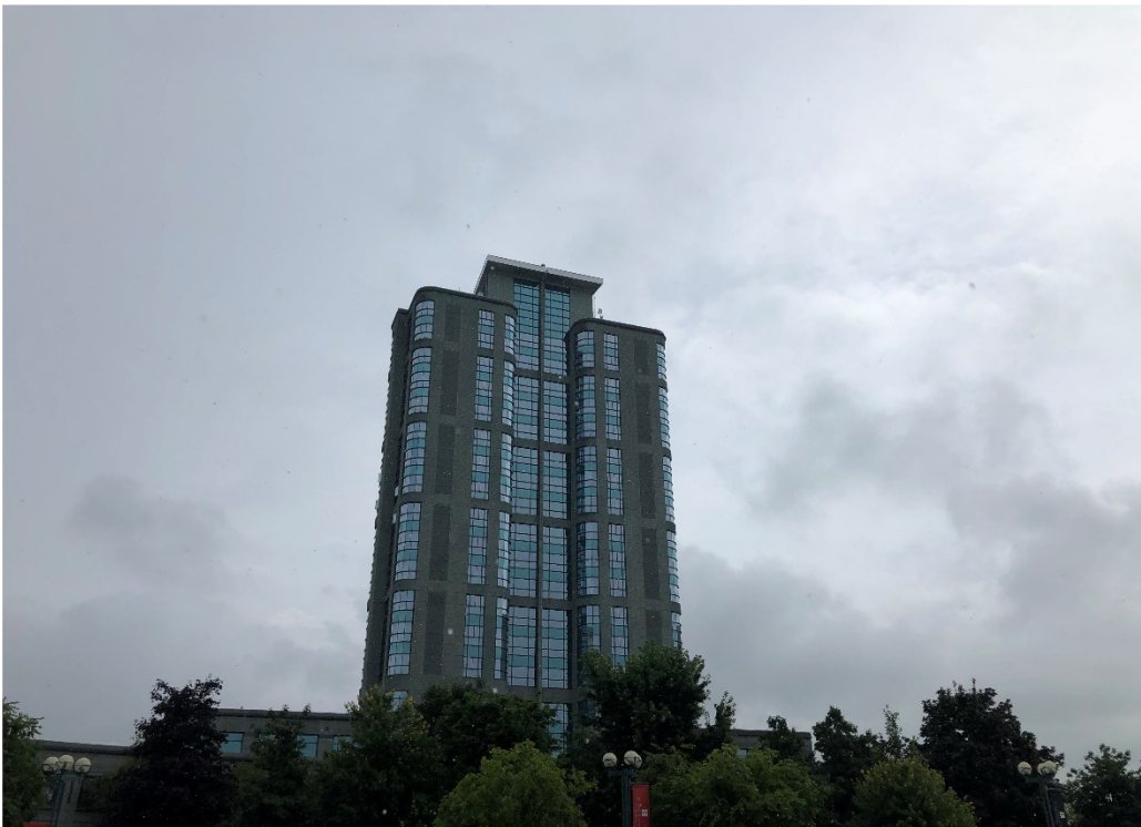
Photograph 8: View to the east of the Phase I Property.
