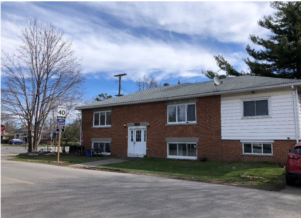
Photograph 6: View looking east from Edith Avenue, towards 304 Donald Street.
