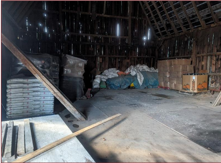
Photograph L5 – Looking south and the inside view of Structure 1 (Two Storey Barn).
