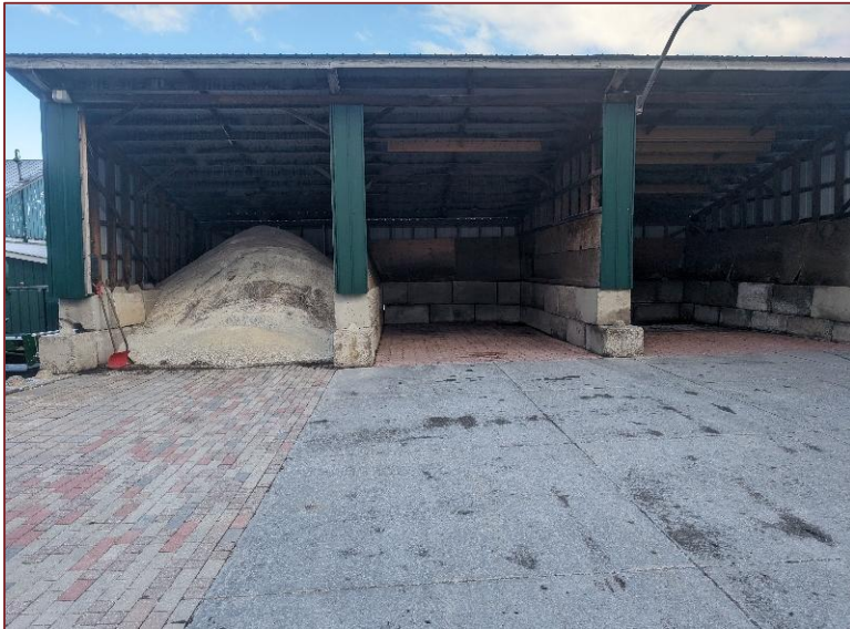
Photograph L19 – Looking north towards Structure 9 (Salt Storage).
