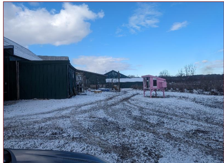
Photograph L4 – Looking west. Chicken coops and the area behind Structure 4 (Material Storage), Structure 5 (Material Storage), Structure 9 (Salt Storage) and Structure 3 (Material Storage in the background).
