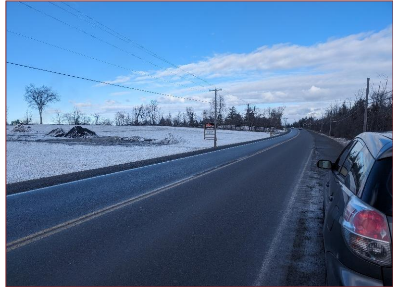
Photograph L2 – Looking north along the Rideau Valley Drive. The Site is to the left of the Rideau Valley Drive. Roadside drainage ditches are located on both sides of the Rideau Valley Drive.
