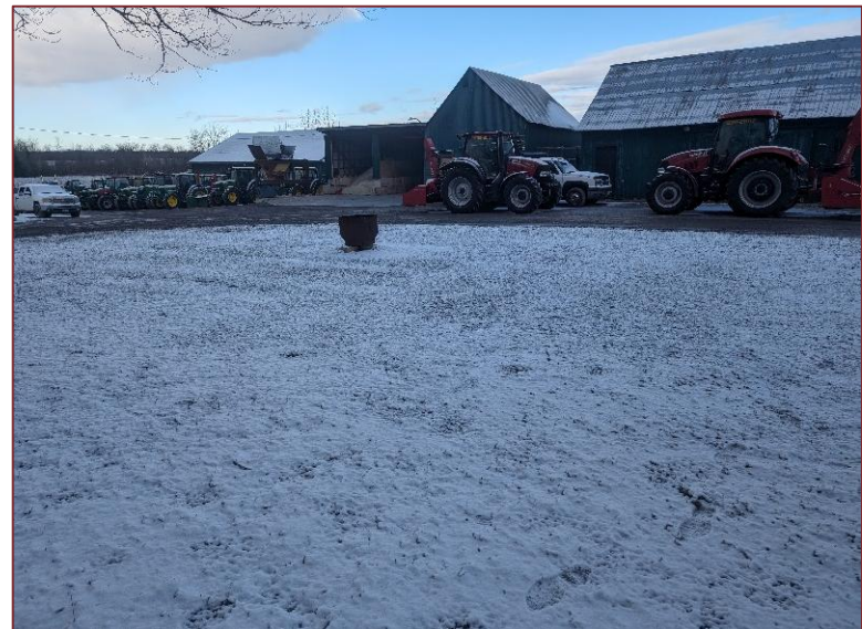
Photograph L24 – Looking northwest. From left to right is Structure 3 (Material Storage), Structure 9 (Salt Storage), Structure 5 (Material Storage), and Structure 4 (Material Storage).
