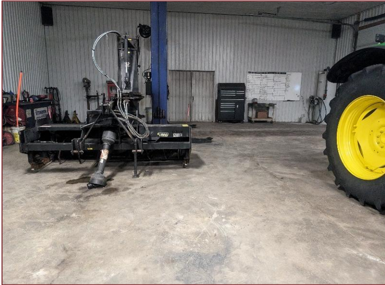
Photograph L13 – Looking west inside the Structure 7 (Building Workshop). A photo of the hydraulic lift.
