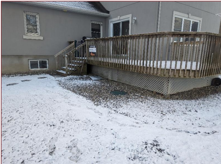
Photograph L23 – Looking south towards Structure 2 (Office Building). A septic tank can be seen in front of the Office Building.
