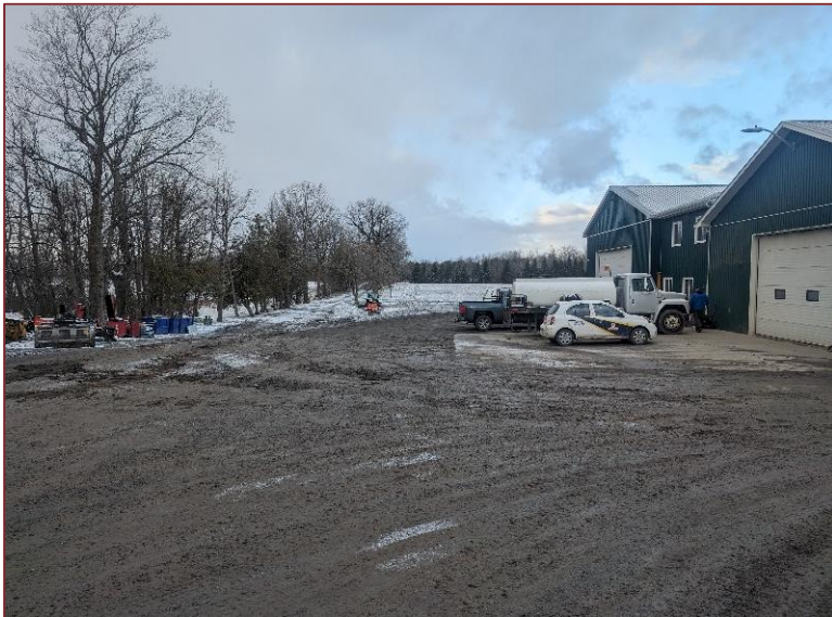
Photograph L7 – Looking west. Structure 7 (Building Workshop) with the bay doors can be seen to the right.
