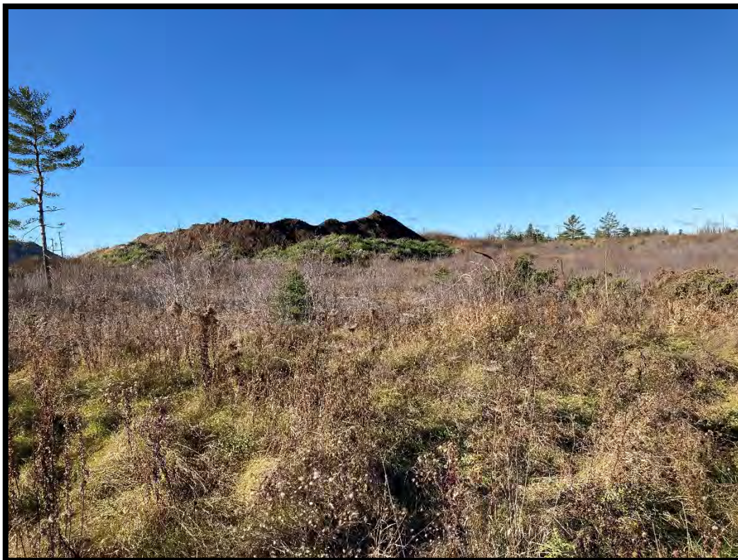
Figure 2: Uneven ground of stone fill, piles in background, north-eastern portion. (MH1141-D010)
