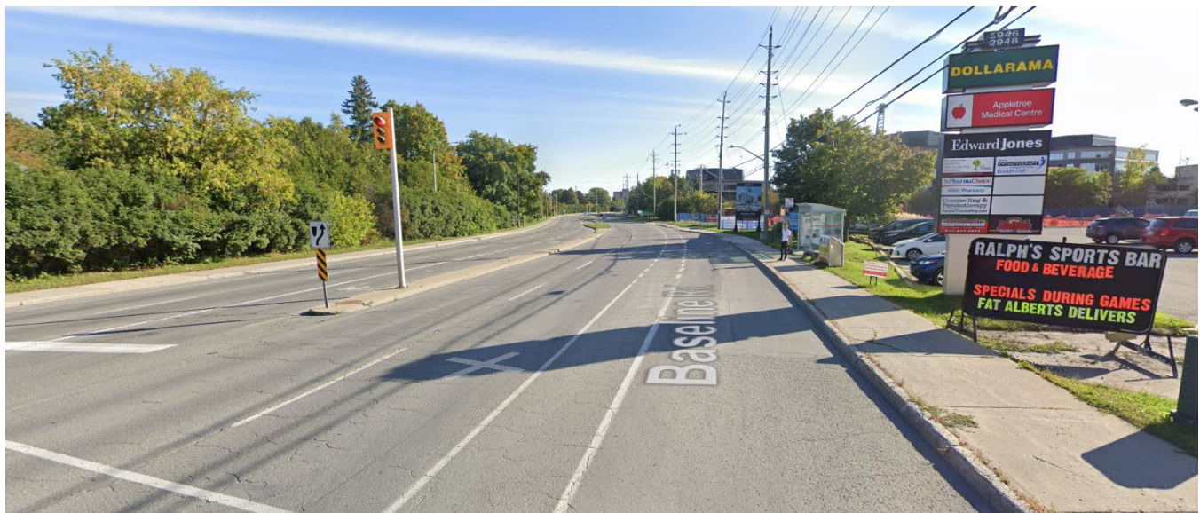
Figure 8 Existing Painted Bicycle Lane along Baseline Road.
