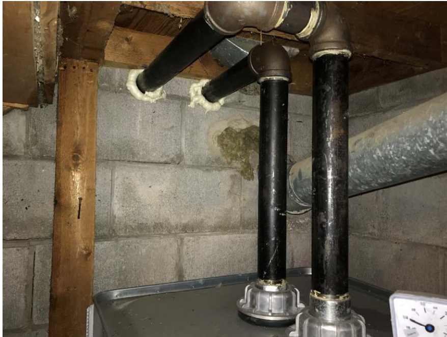
Photograph 29: Heating oil tank, fill and vent lines
