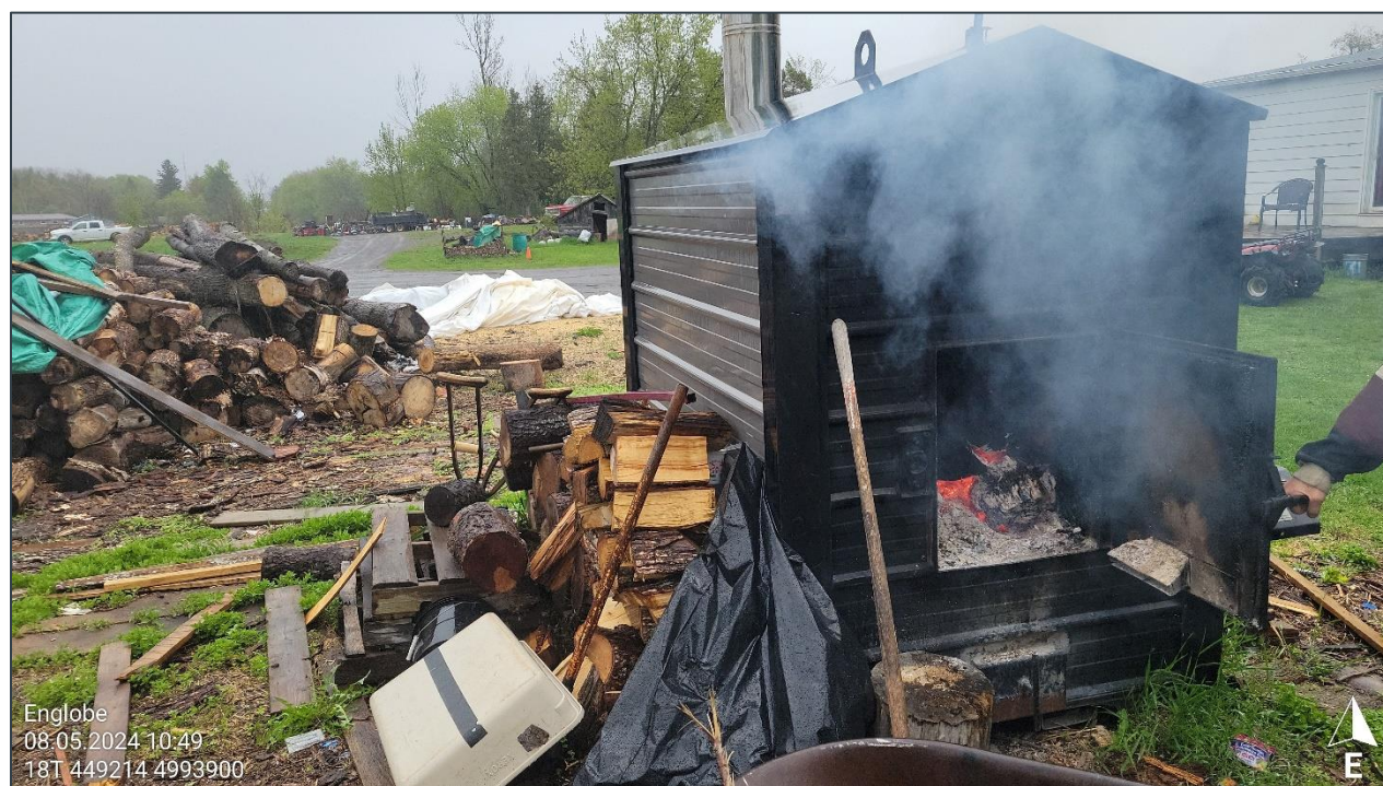
Photograph 8: Exterior wood burning stove
