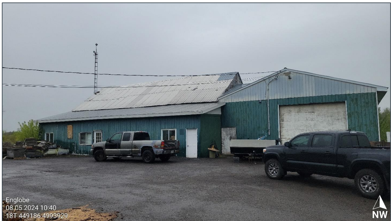
Photograph 4: Commercial service garage
