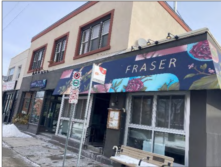
Photo 1 – West elevation of the Site Building A, looking northeast.
