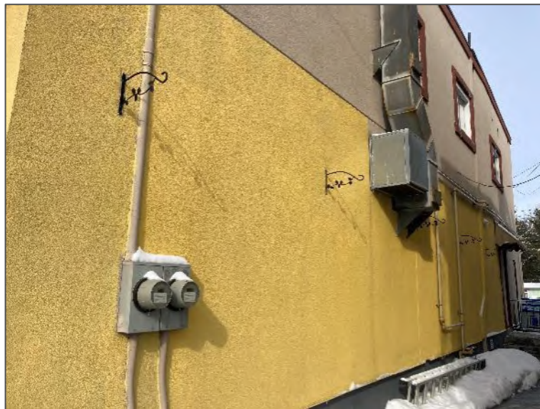
Photo 8 – East elevation of Site Building C, looking north.
