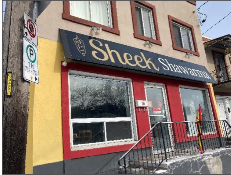
Photo 7 – South elevation of Site Building C, looking northeast.
