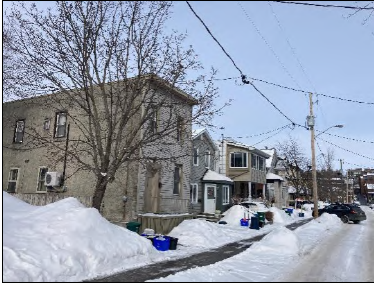
Photo 13 – Looking south along Douglas Avenue.
