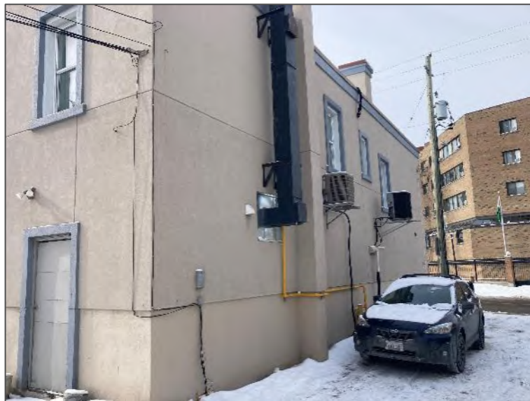
Photo 6 – North elevation of the Site Building B, looking southwest.
