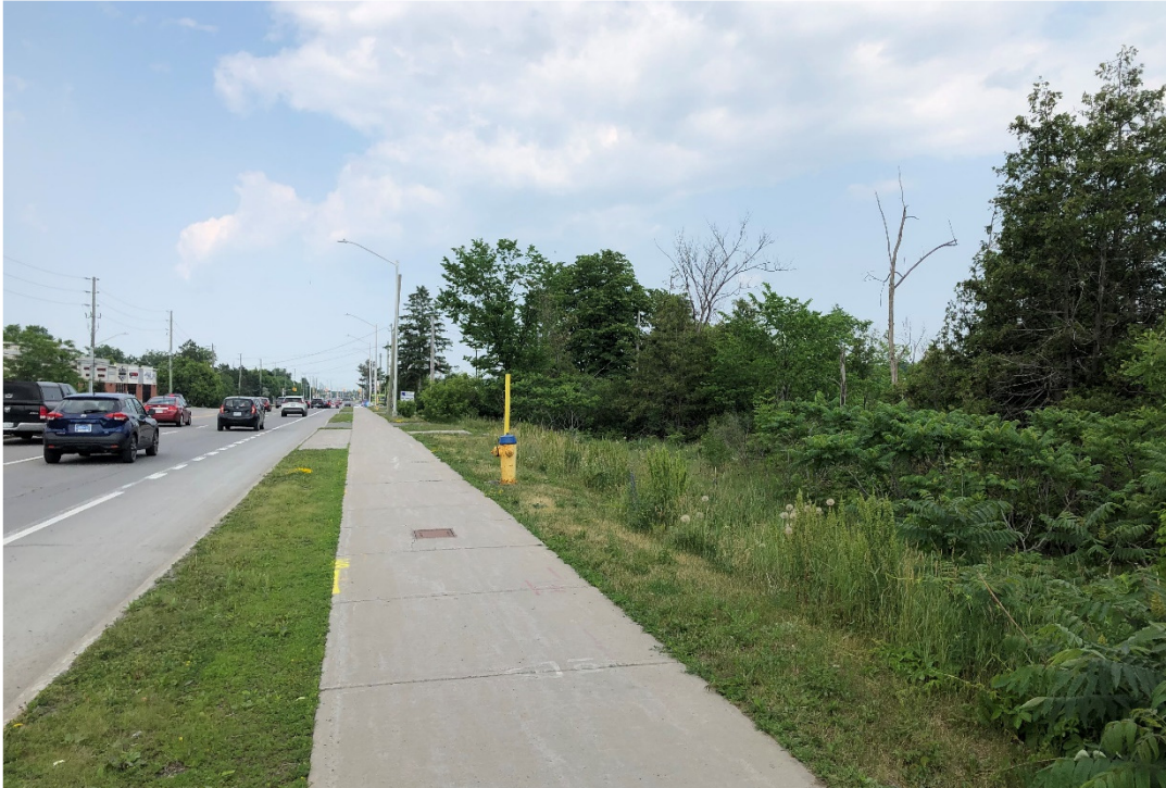
Photograph 5: View to the east of the Phase I Property from Innes Road.
